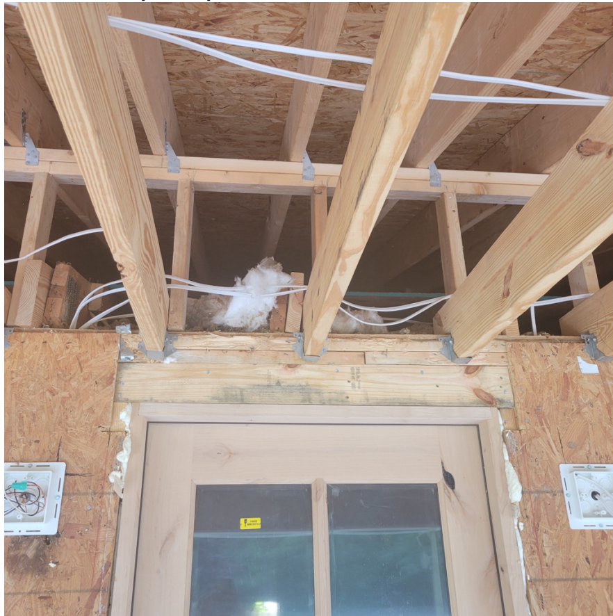
Figure 1 – Ceiling joists notched and installed with hangers and front door header
