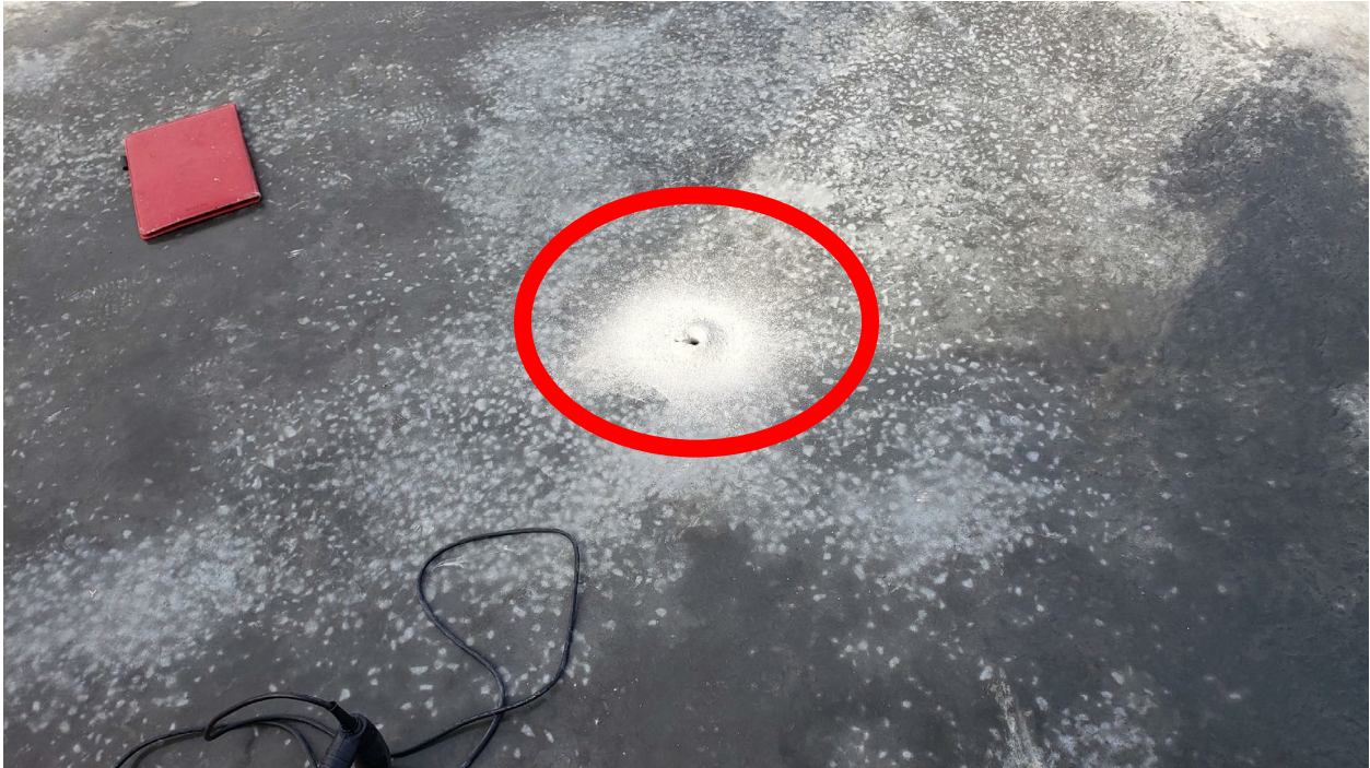
Slab inspected and examples of areas drilled
