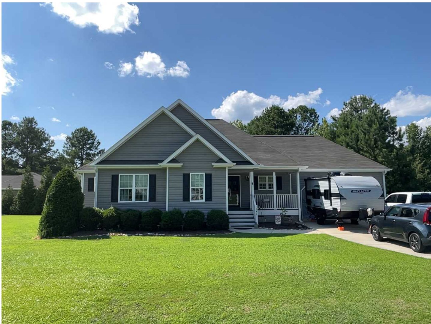
1 Main Level - 5-Front Elevation Date Taken: 7/11/2023
