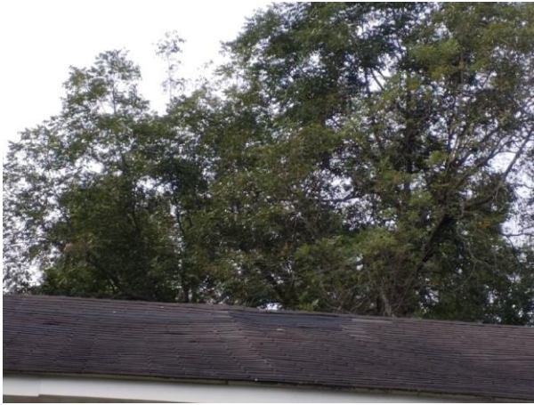
001A, 001 - Roofing, Composite Shingle, Side A, Main Floor
