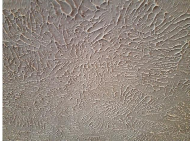
003A, 003 - Gypsum Wallboard Surface Texture/Skim Coat, Living Room, Main Floor
