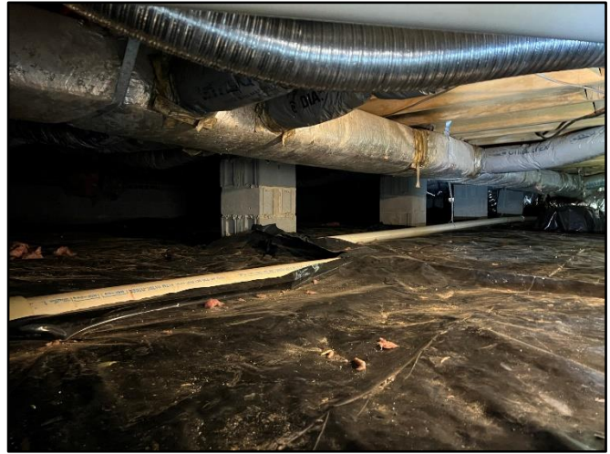
Photo 2 Existing vapor retarder and overall crawlspace.
