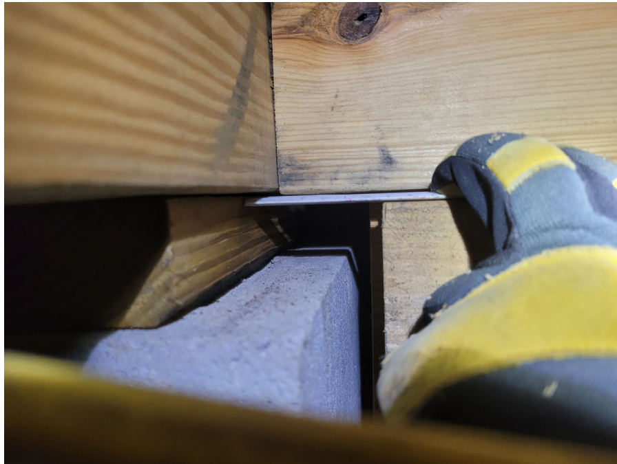
Picture 5 – Example of girder set low to perimeter sill plate
