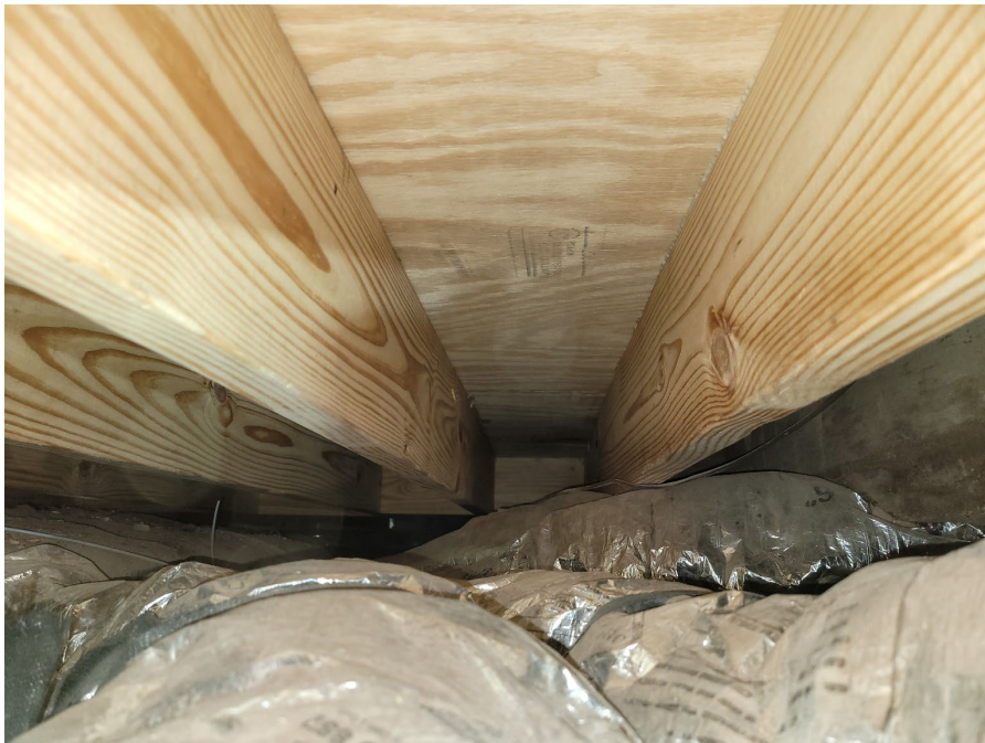
Picture 2 – Example of new floor joists and subfloor
