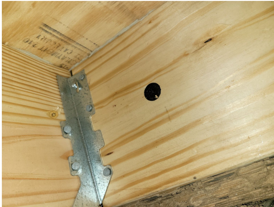
Picture 3 – Example of joist hangers and structural wood screws
