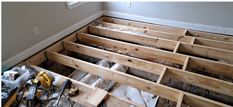
Picture 4 – Photographic evidence repair in progress
