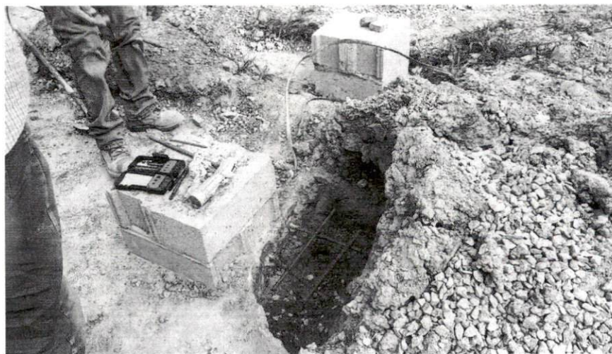
Examples of foundation constructed and footing projection repair made
