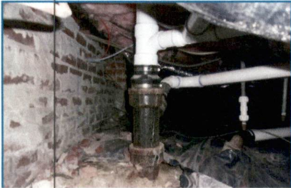
P15. Common Cast Iron Drain
