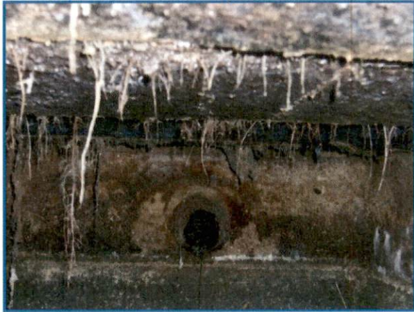
P8. Septic Tank Outlet Interior
