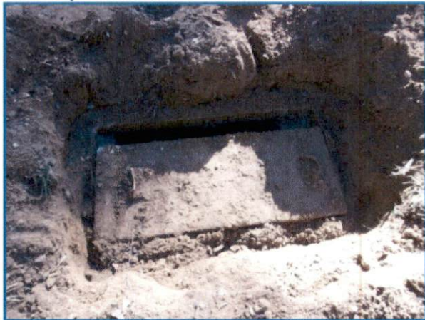
P4. Septic Tank Outlet Slab
