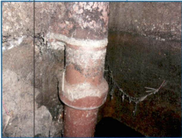
P7. Septic Tank Outlet Sanitary Tee
