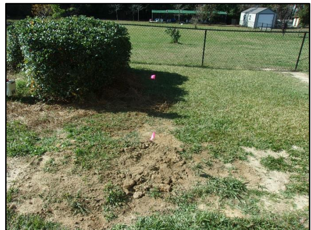
Re-covered Access Openings:
