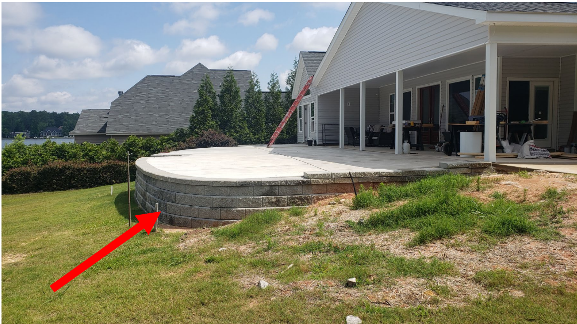
Retaining wall inspected and wall drains to be installed
