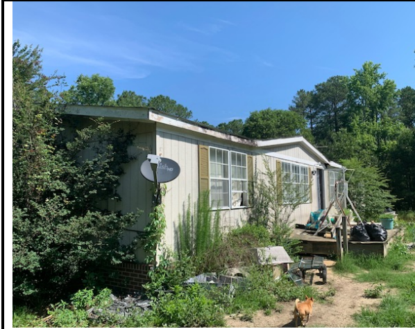
Front of Residence & Roofing Shingles
