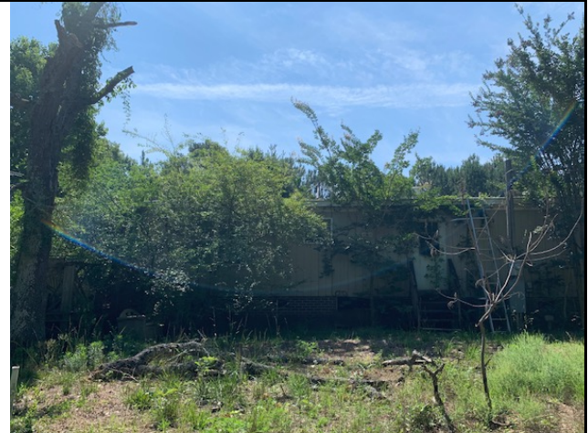
Back of Residence
