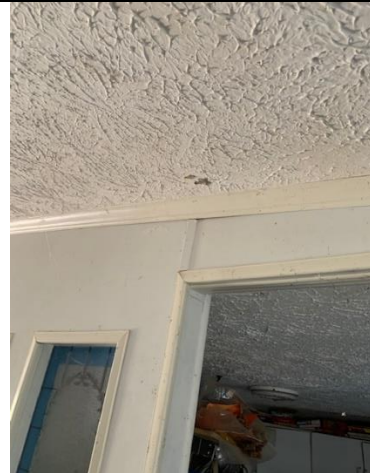
Textured Ceiling – Negative for Asbestos
