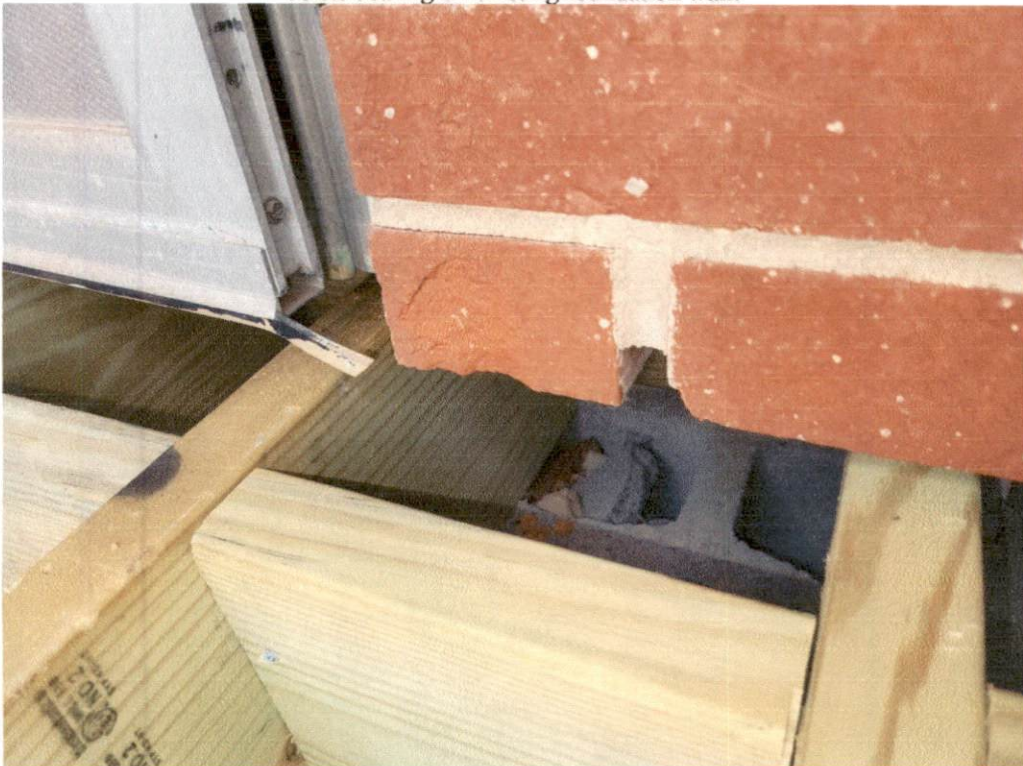
Joists bearing on existing foundation wall:
