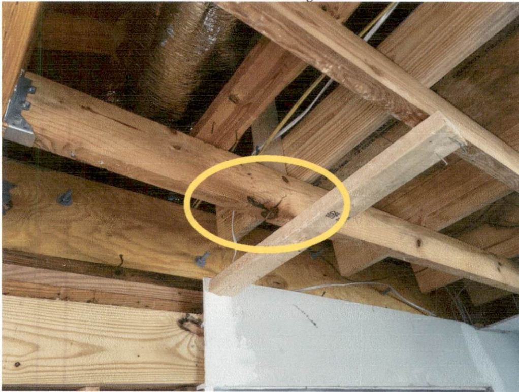
Item 2: Damaged rafter with blocking
