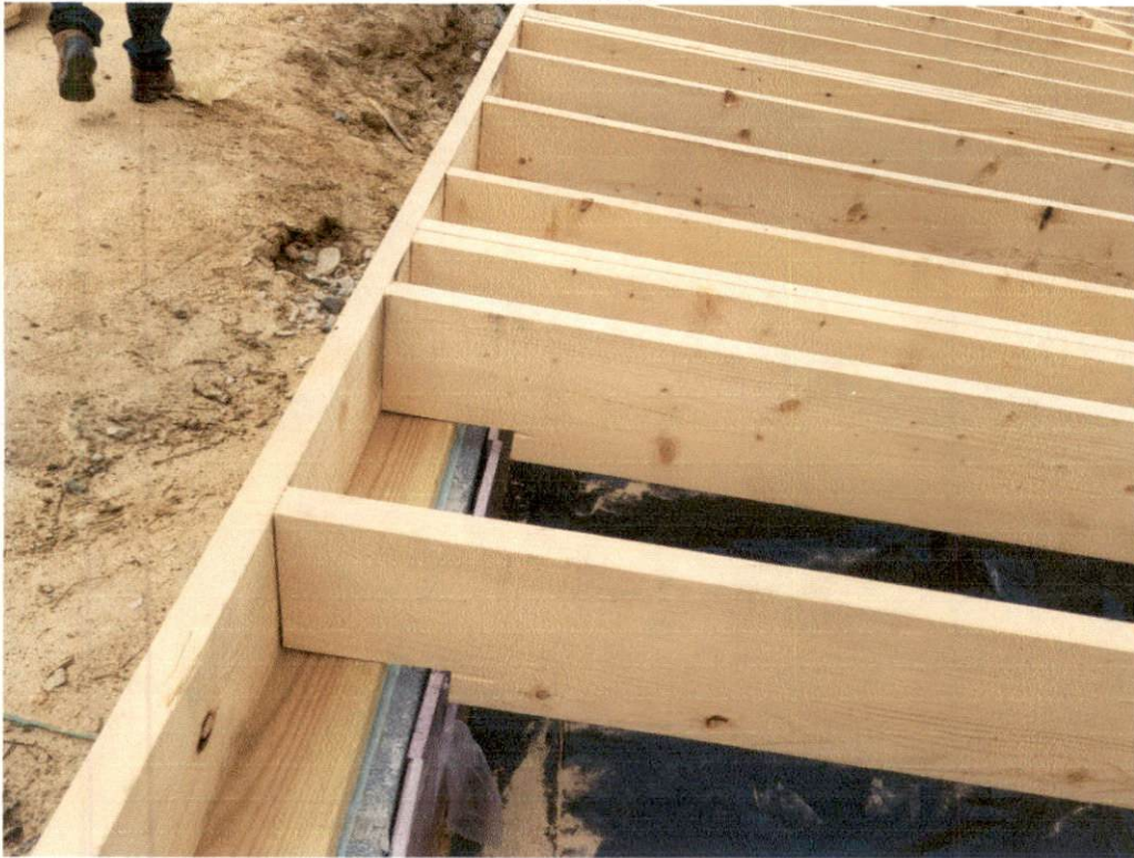
Joists bearing on existing foundation wall:
