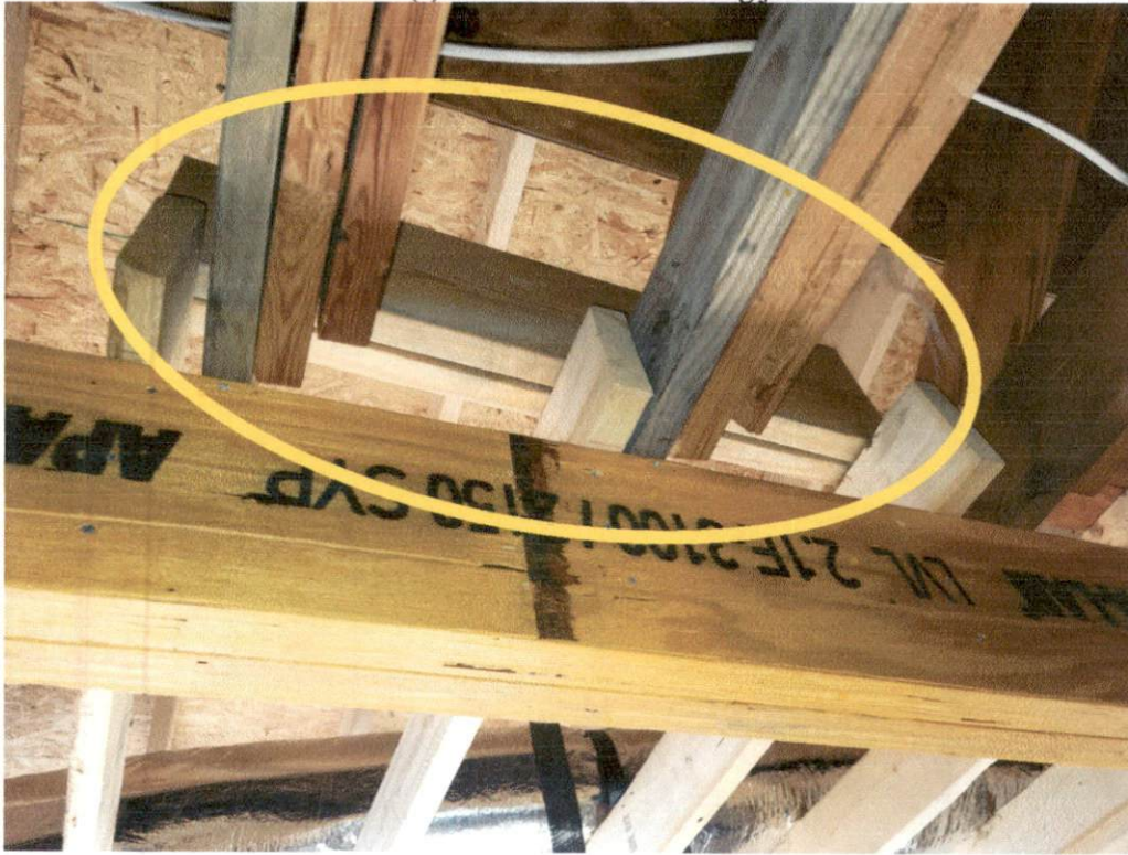
Item 3: (2) 2 x 10 installed on ceiling joists
