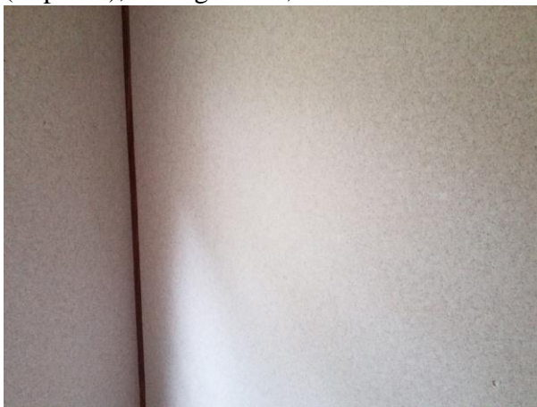
003A, 003 - Gypsum Wallboard, Bedroom 3, Main floor
