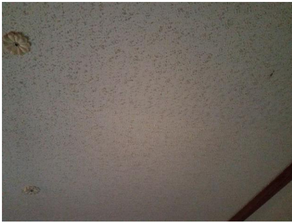
001A, 001 - Textured Ceiling Material (Popcorn), Living Room, Main floor
