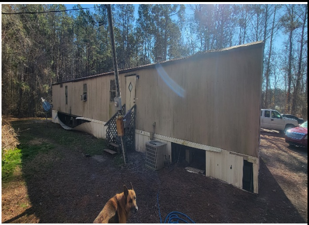
Rear of Residence, Viewed from Street Level
