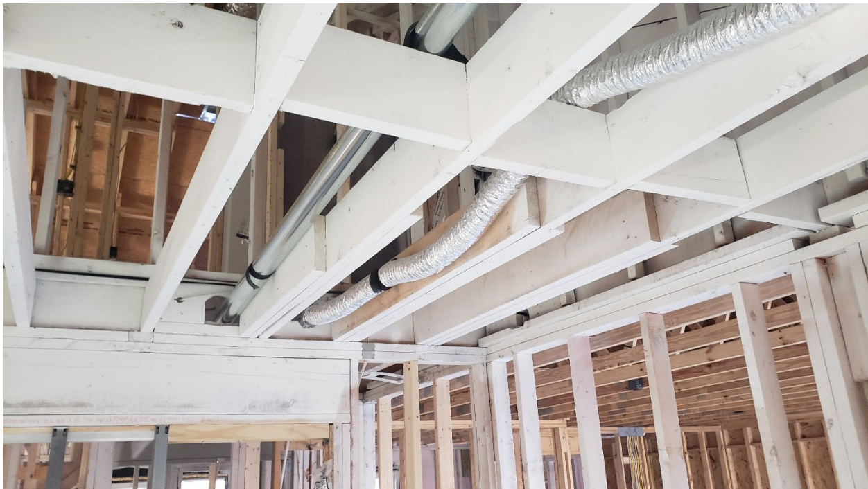
“Scabbed” Ceiling Joists
