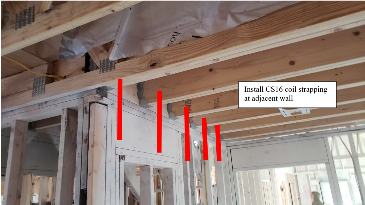
“Scabbed” Ceiling Joists
