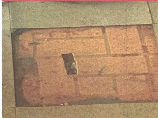
(8A,8B) – Sheetgood (Brown) Chrysotile 20%/ Mastic 2% & Floor Tile (Tan) 5%
