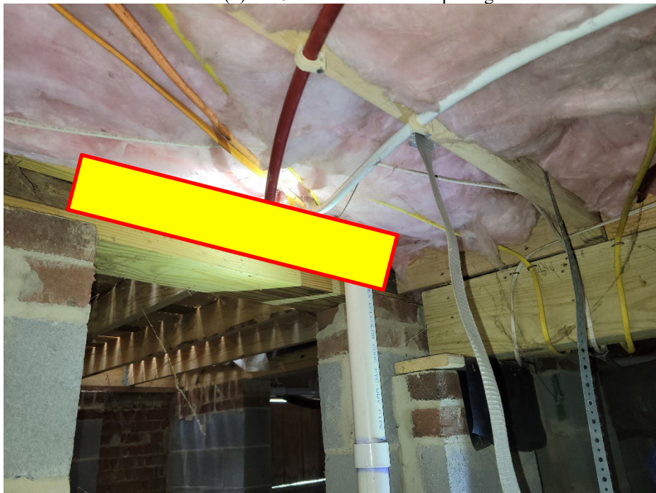
Install (2) 2 x 8 header over crawl opening
