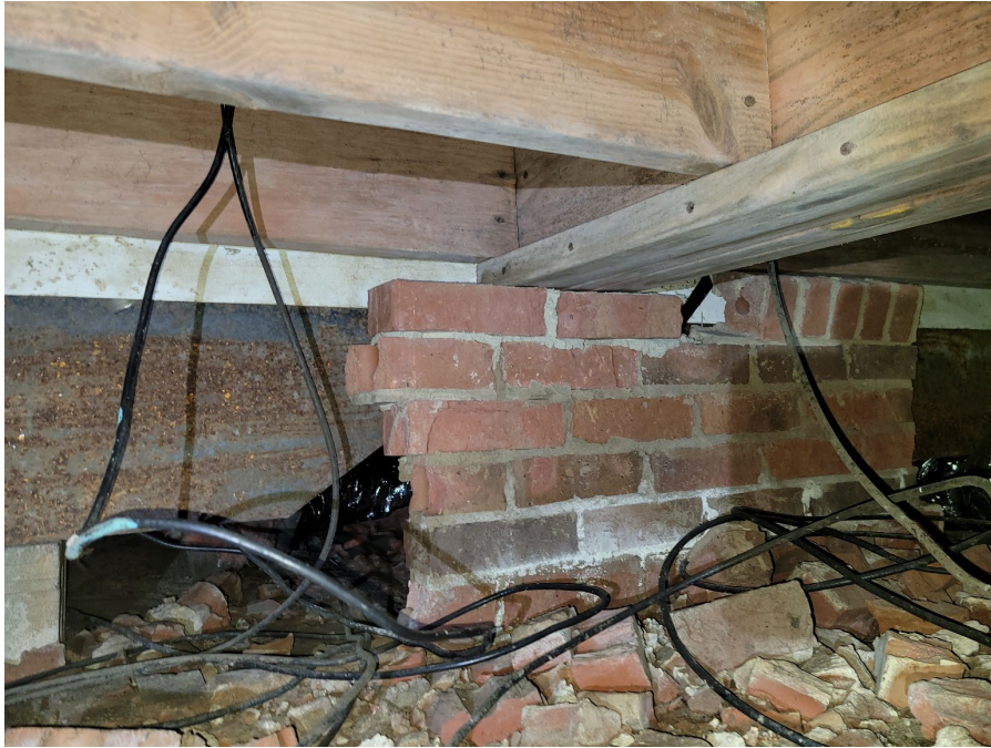
Picture 11– Example of girder end bearing on the curtain wall
