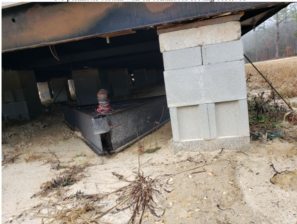
No perimeter curtain wall on continuous footing observed
