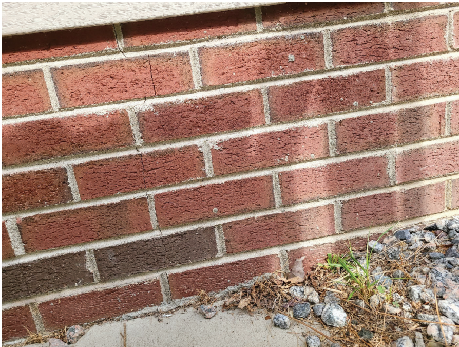
Picture 2 – Foundation crack
