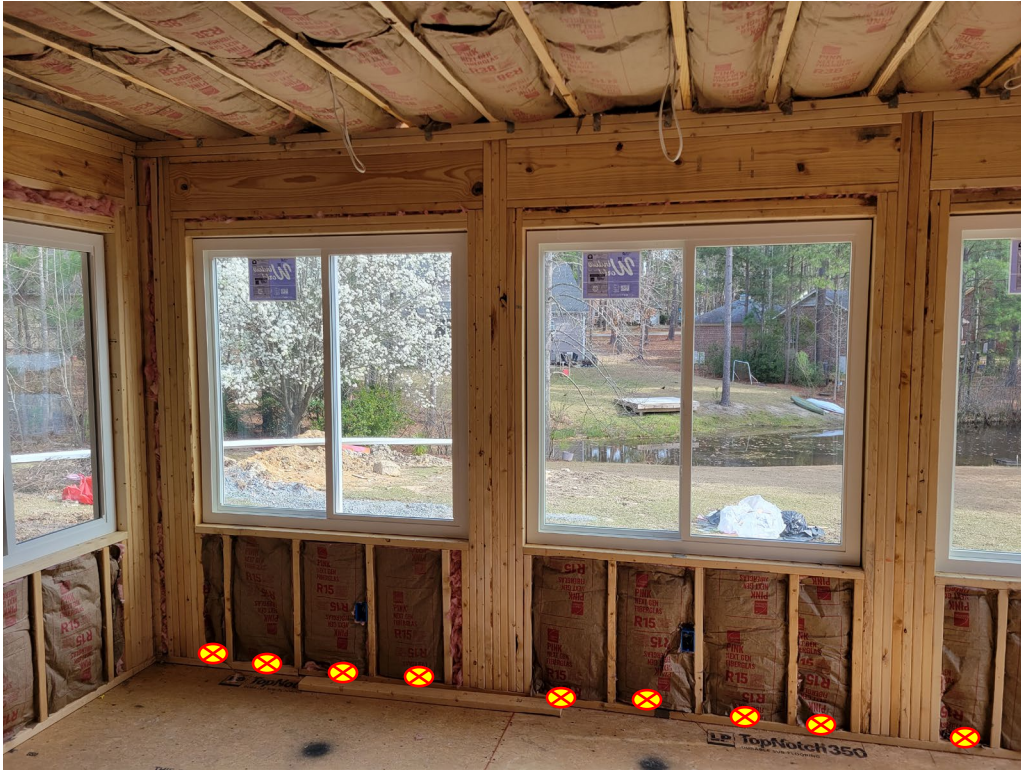
Item 1.b. Install additional 2 x 4 studs packed tightly to corners
