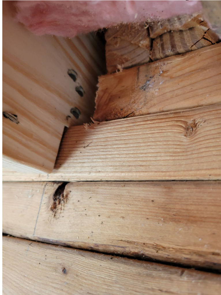
Item 2. Install 2 x 8 x 1' scabs for addition bearing.
