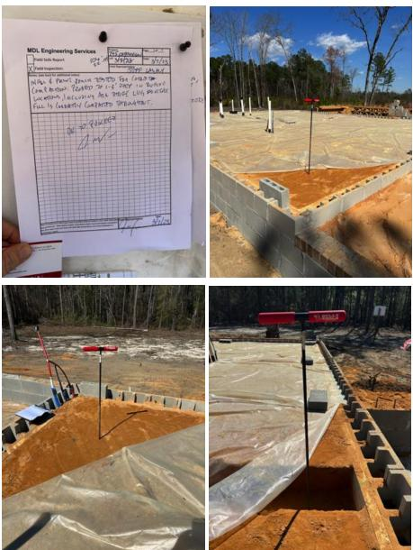
MDL Engineering was contacted on March 6, 2023 to re-test for compaction. The material was again probed with a ½" rod and/or use of a DCP technique to correlate surface soil conditions with bearing capacity. This test was performed in six different locations in the field and in multiple locations in every lug footing. The material passed the compaction in every spot. In addition, there was no visible sign of organic materials present this time.
