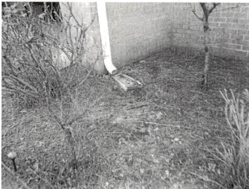
Picture 8 – Example of roof gutter downspout installed for discharge at foundation
