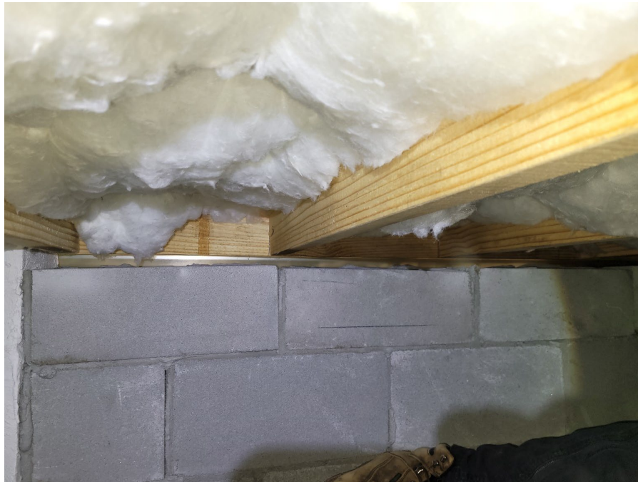
Picture 3 – New rim band out of contact over new foundation wall
