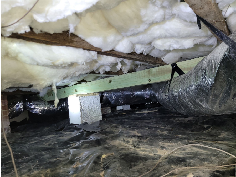
Picture 5 – New 6x6 girder supported by CMU pier
