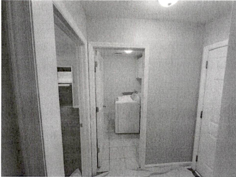
Item #3: Wall to be Removed
