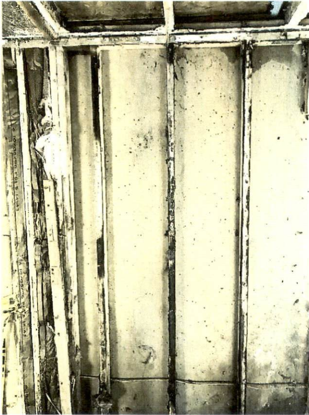
Figure 2. Representation of some of the burned members
