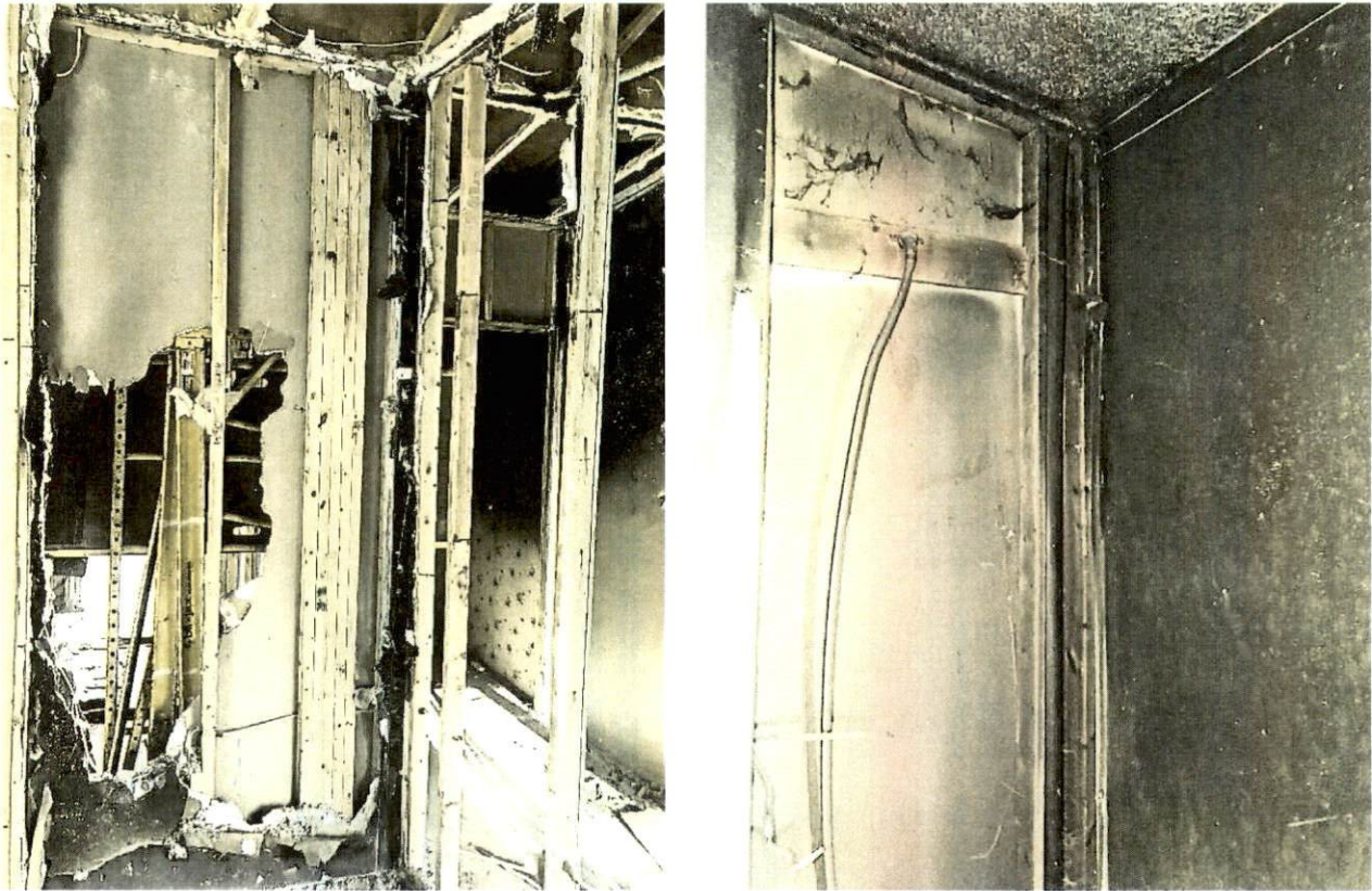
Figure 2. Representation of some of the burned members
