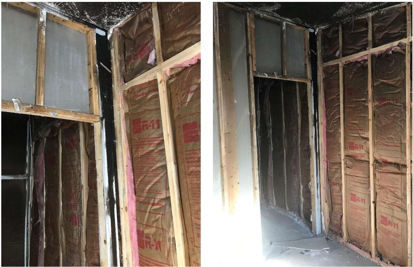
Figure 2. Representation of some of the burned members
