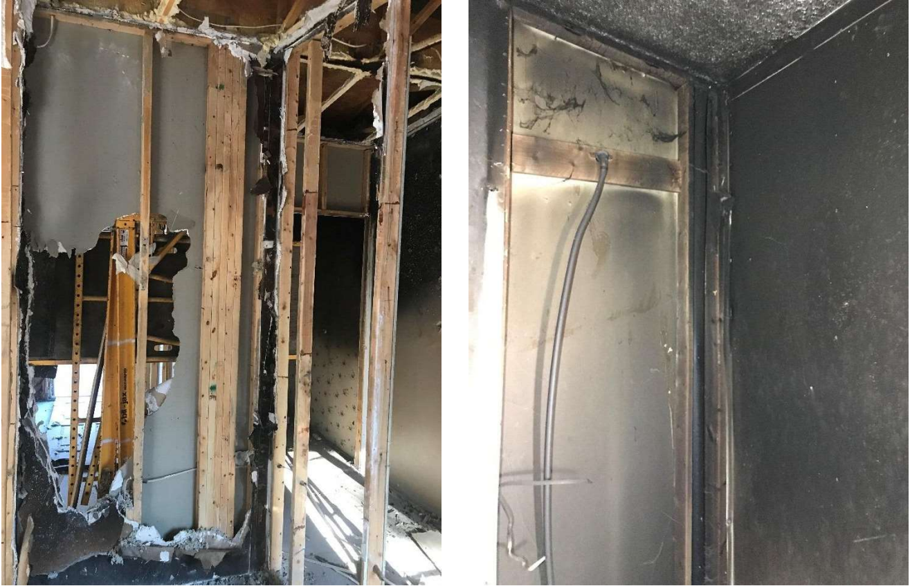
Figure 2. Representation of some of the burned members
