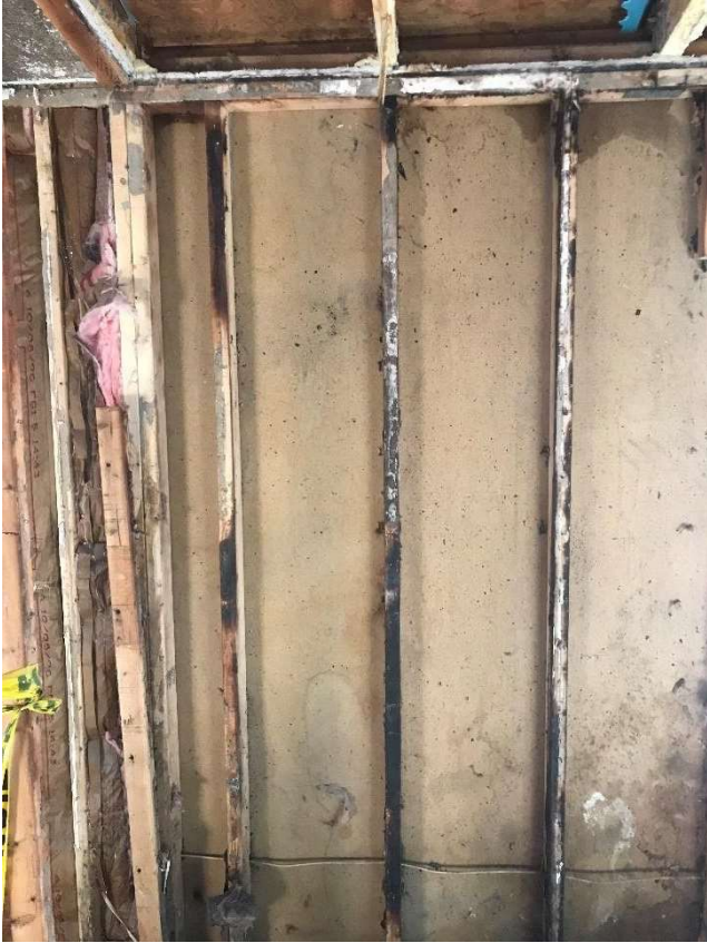
Figure 2. Representation of some of the burned members
