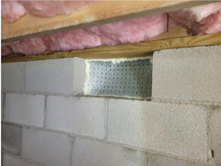
Picture 7 – Example of sealed crawlspace vents
