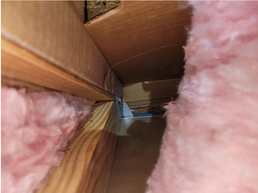
Picture 3 –Example of “H2.5A” hurricane tie
