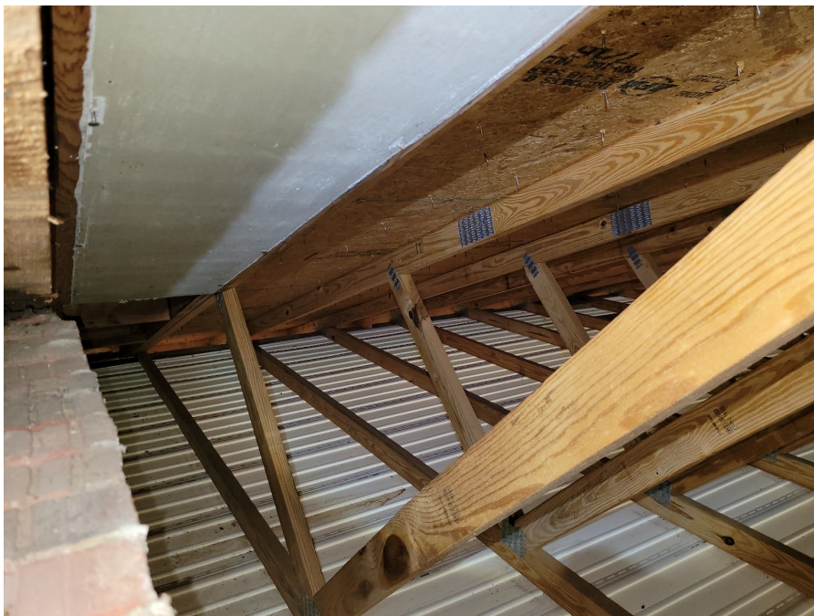
Picture 2 – Example of roof trusses over the addition and carport
