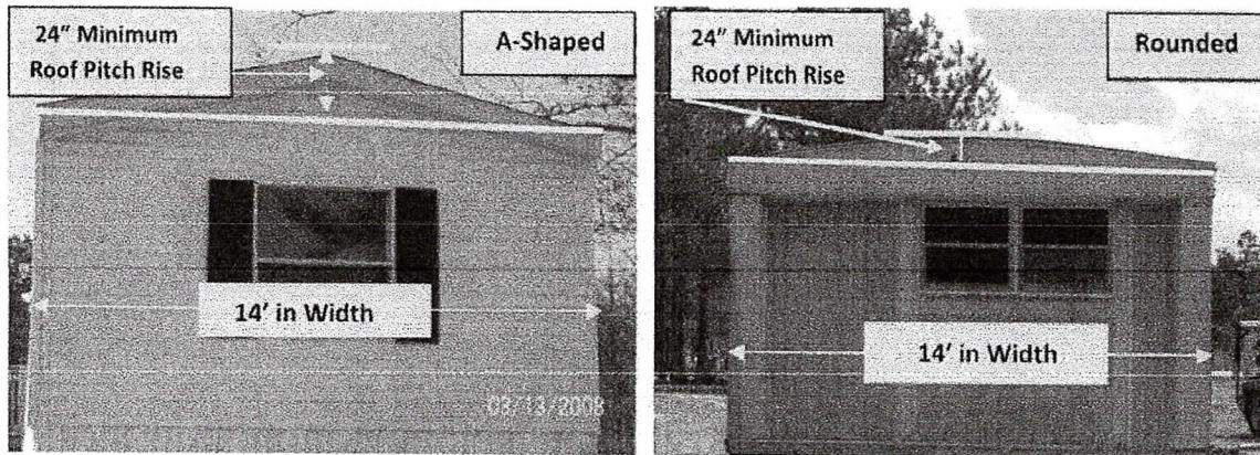
Note: Most Rounded Roofs Will Not Meet The Roof Pitch Requirement As Illustrated. The Measurement From The Peak Of The Roof To The Base Line Of The Roof Must Be 12" For Every 7' Of Total Width Of The Home. (Ex: 14' Wide Home = 24" Roof Rise)
