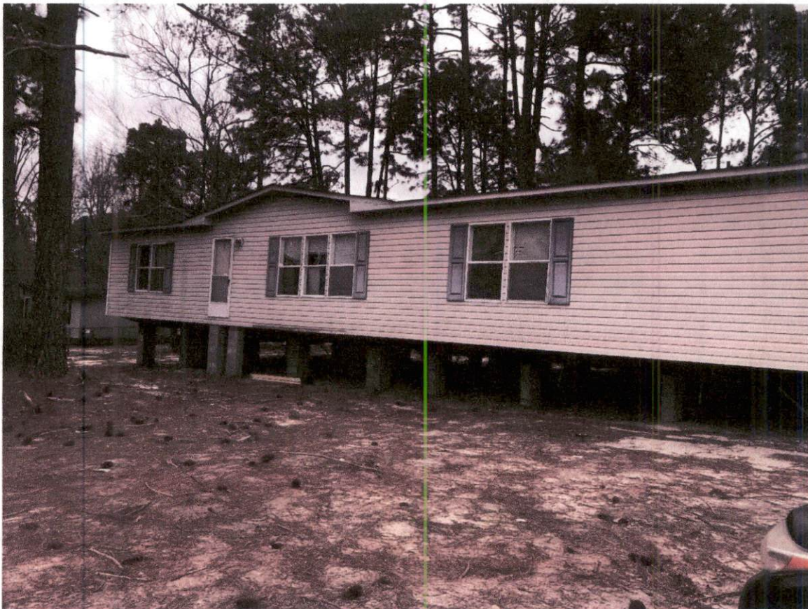
Figure 1. Main entrance of the house facing South (towards Old Dutch Rd)
