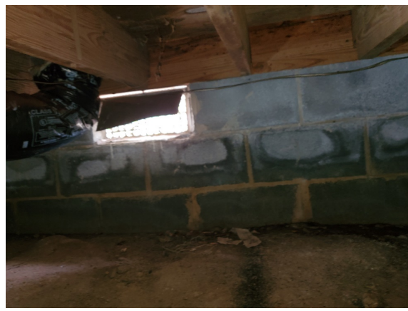
Picture 10 – Example of curtain wall without pilasters
