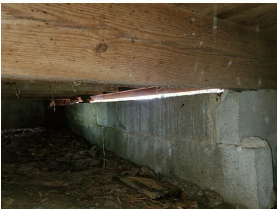
Picture 11 – Rim out of contact with pilasters and curtain wall
