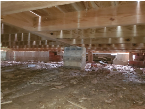
Picture 15 – Dry-stacked pier
