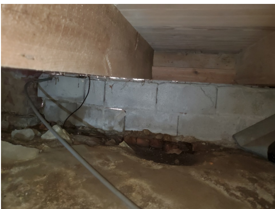
Picture 5 – Example of cracks in curtain wall
