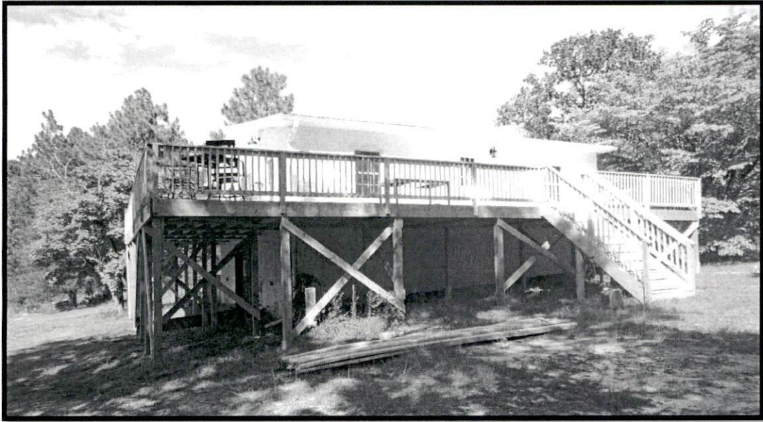
Photo #1 - This is an overall photo of the deck.
