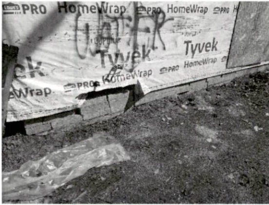
Example of Dry Stacked Foundation Wall
