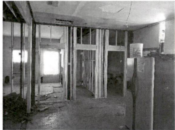
Example of Interior (2) 2 x 10 Door Headers
