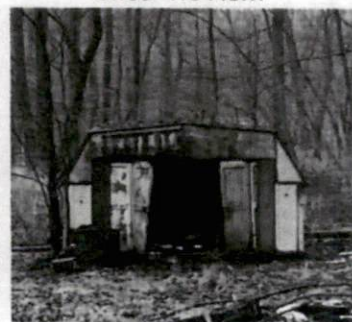
Shed -No ACM
