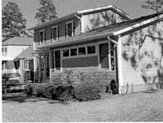
Picture 2 – Back office window to be modified
