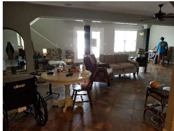
Picture 4 – Posts and dropped beam
