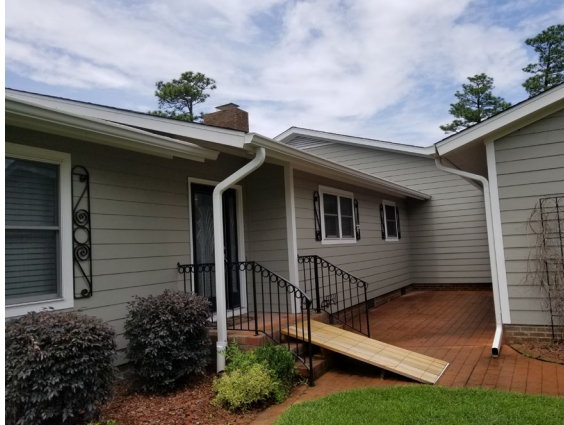
Picture 2 – Front kitchen window to be widened (at right of picture)
