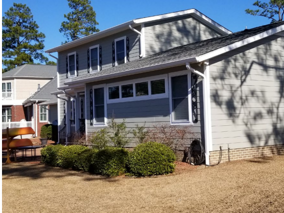
Picture 2 – Back office window to be modified
