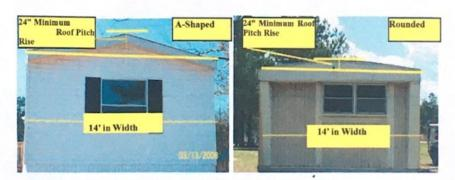
Note: Most Rounded Roofs Will Not Meet The Roof Pitch Requirement As Illustrated. The Measurement From The Peak Of The Roof To The Base Line Of The Roof Must Be 12" For Every 7' Of Total Width Of The Home. (Ex: 14' Wide Home = 24" Roof Rise) Continued.......
