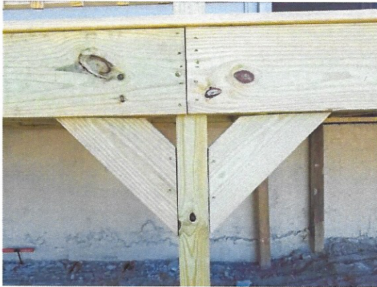
Picture 7 – Example of 2x bracing
