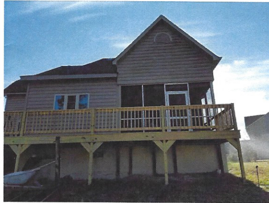
Picture 2 – Example of newly constructed addition at back of home
