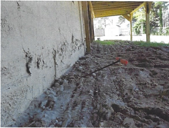
Picture 3 – Example of foundation wall constructed at edge of footing
