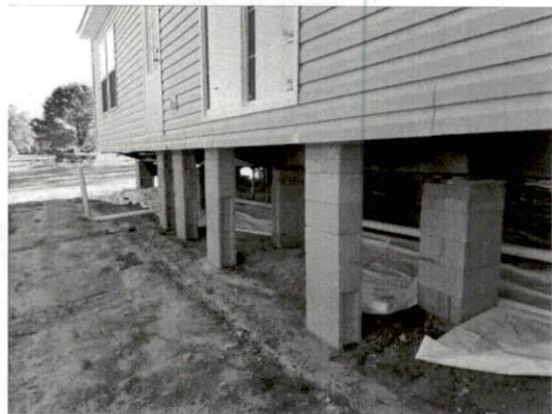
Picture 4 – Example of existing masonry piers
