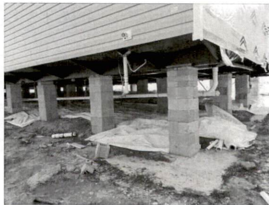
Picture 5 – Example of proposed curtain wall location greater than 40" in height
