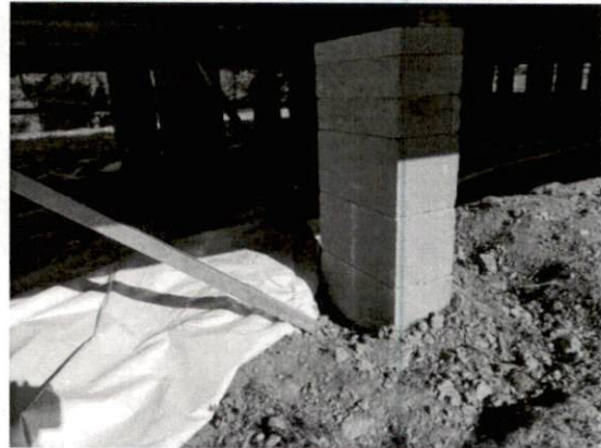
Picture 2 – Existing bracing system
