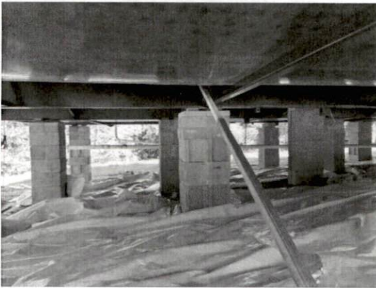
Picture 3 – Existing bracing system
