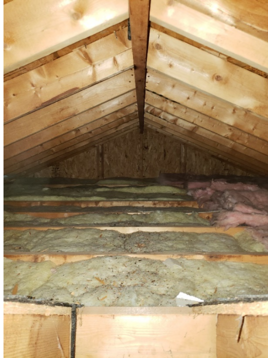
Roof and ceiling framing
