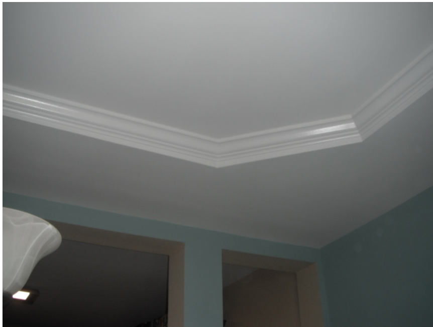
Photograph Number 20 - View of interior ceiling – good condition
