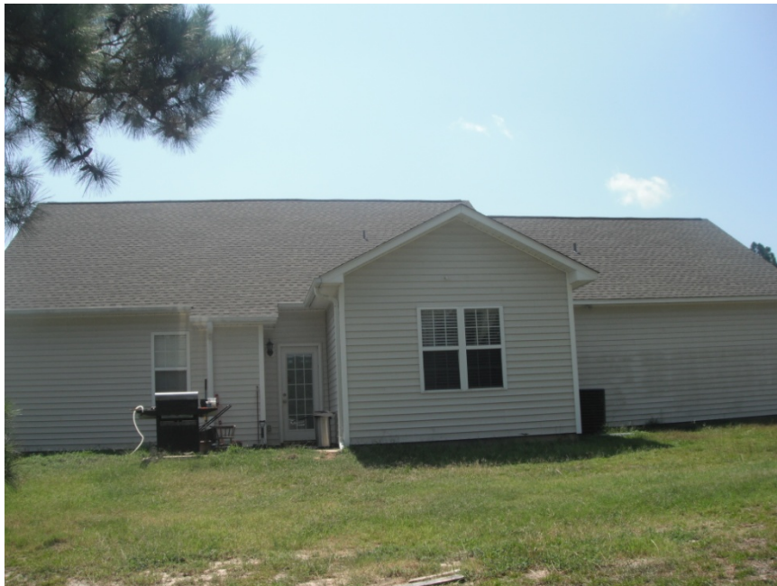
Photograph Number 4 - Rear elevation view.
