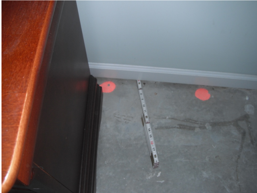
Photograph Number 19 - View of separation between slab and sole plate
