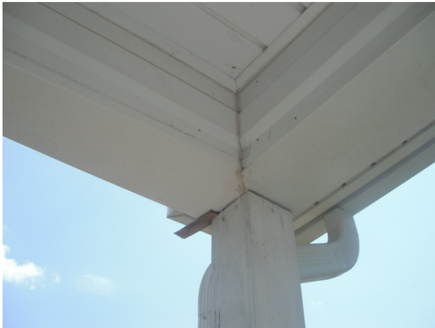
Photograph Number 26 - View of shim at front porch corner post
