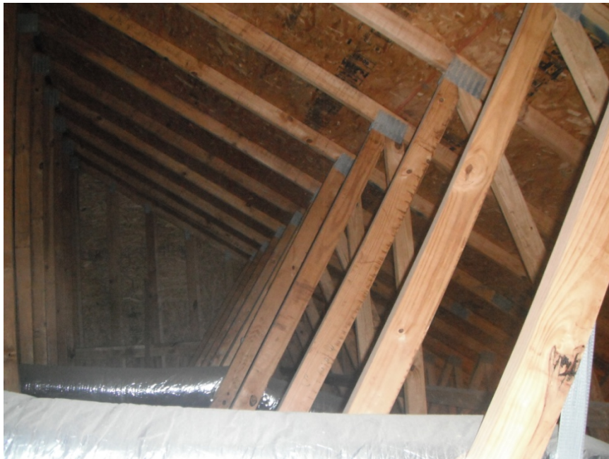
Photograph Number 28 - View of roof trusses – good condition
