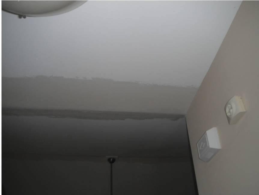
Photograph Number 23 - View of interior drywall repair
