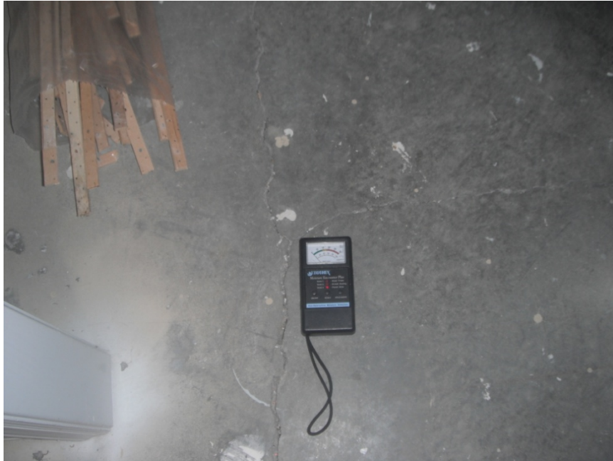
Photograph Number 17 - View of normal moisture reading in slab
