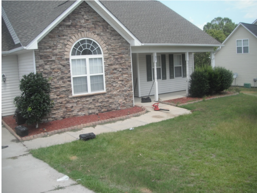
Photograph Number 5 - View of drainage collection area – front yard.
