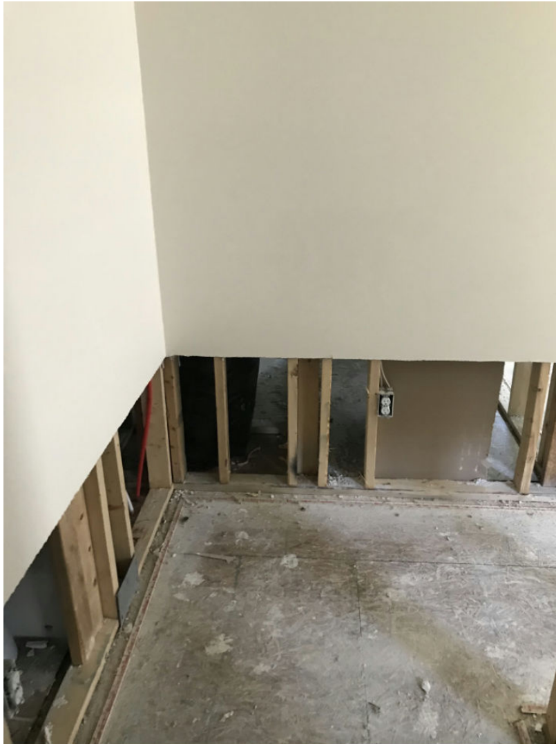
80 Upstairs/Hallway - 89-Hallway2 (3) Date Taken: 7/1/2019
