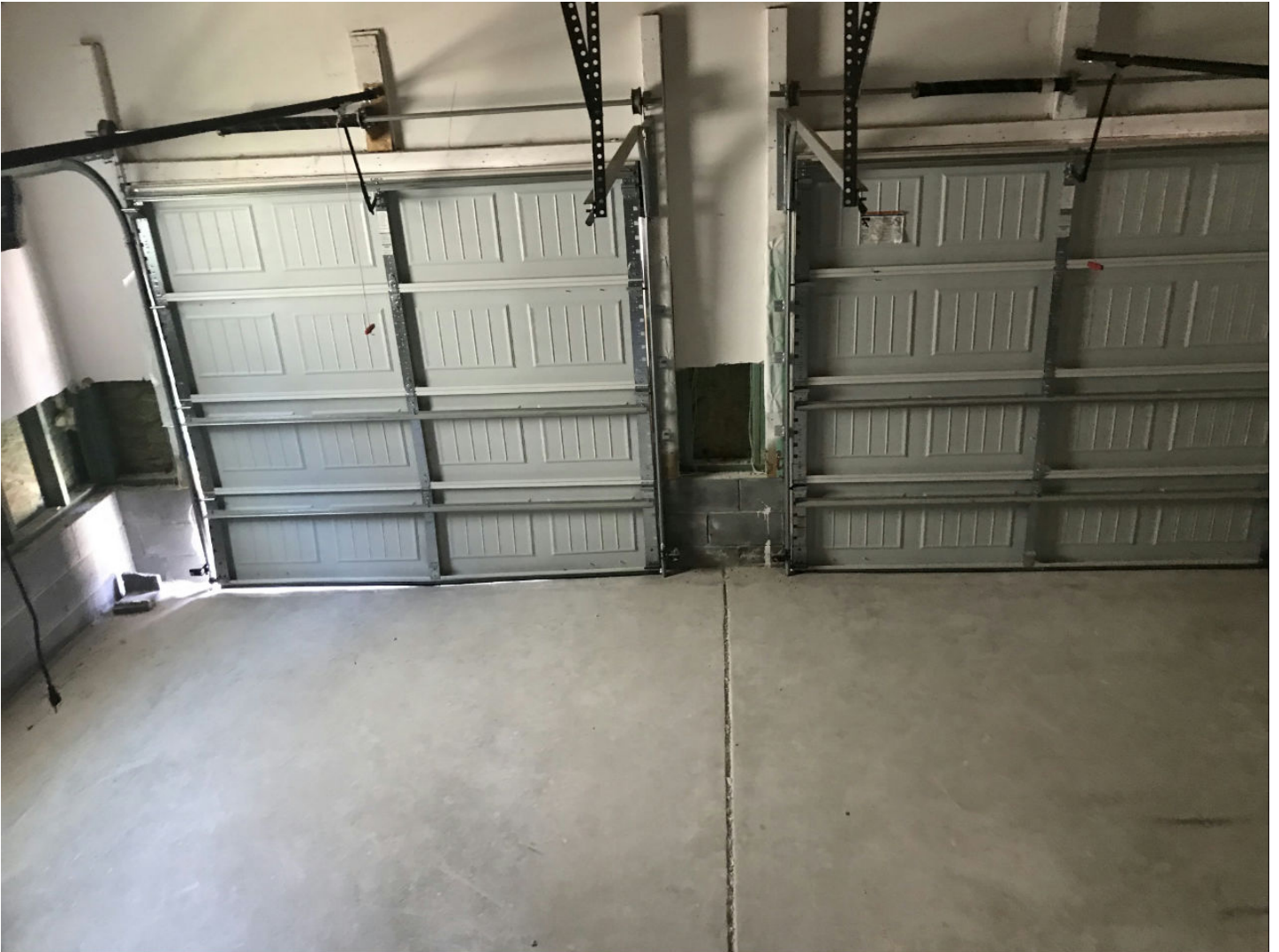
36 Main Level/Garage - 44-Garage (2) Date Taken: 7/1/2019
