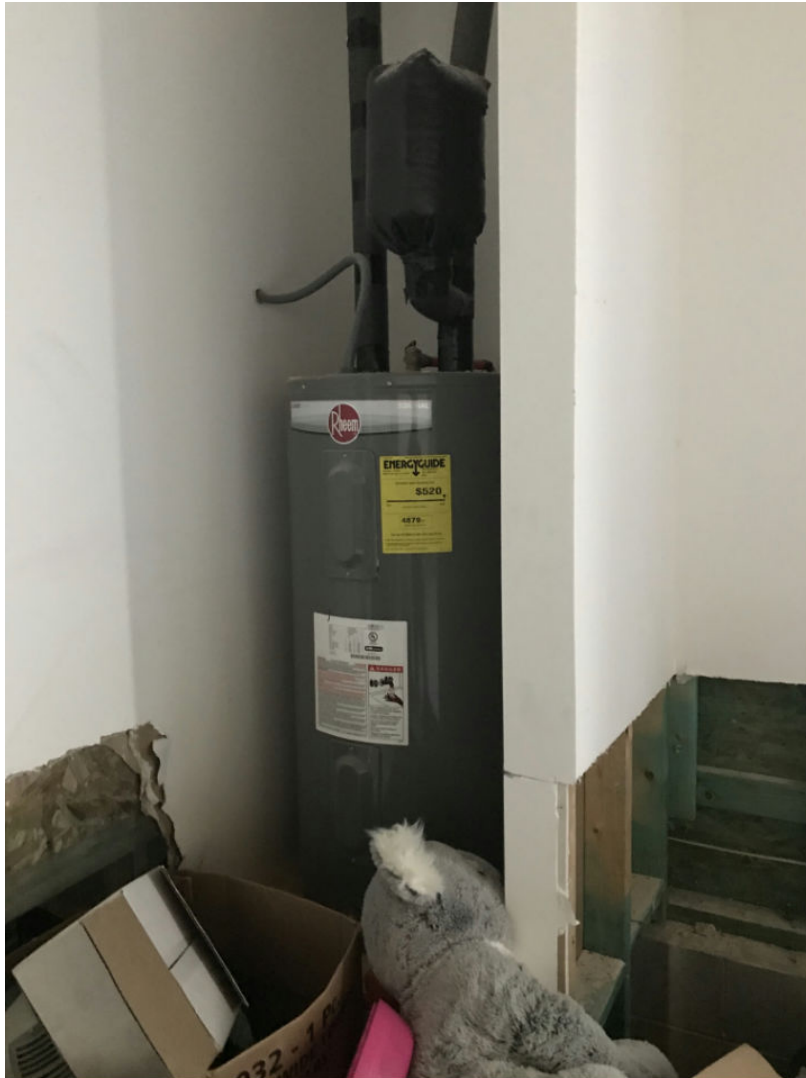
29 Main Level/Garage - 37-Garage (7) Date Taken: 7/1/2019
