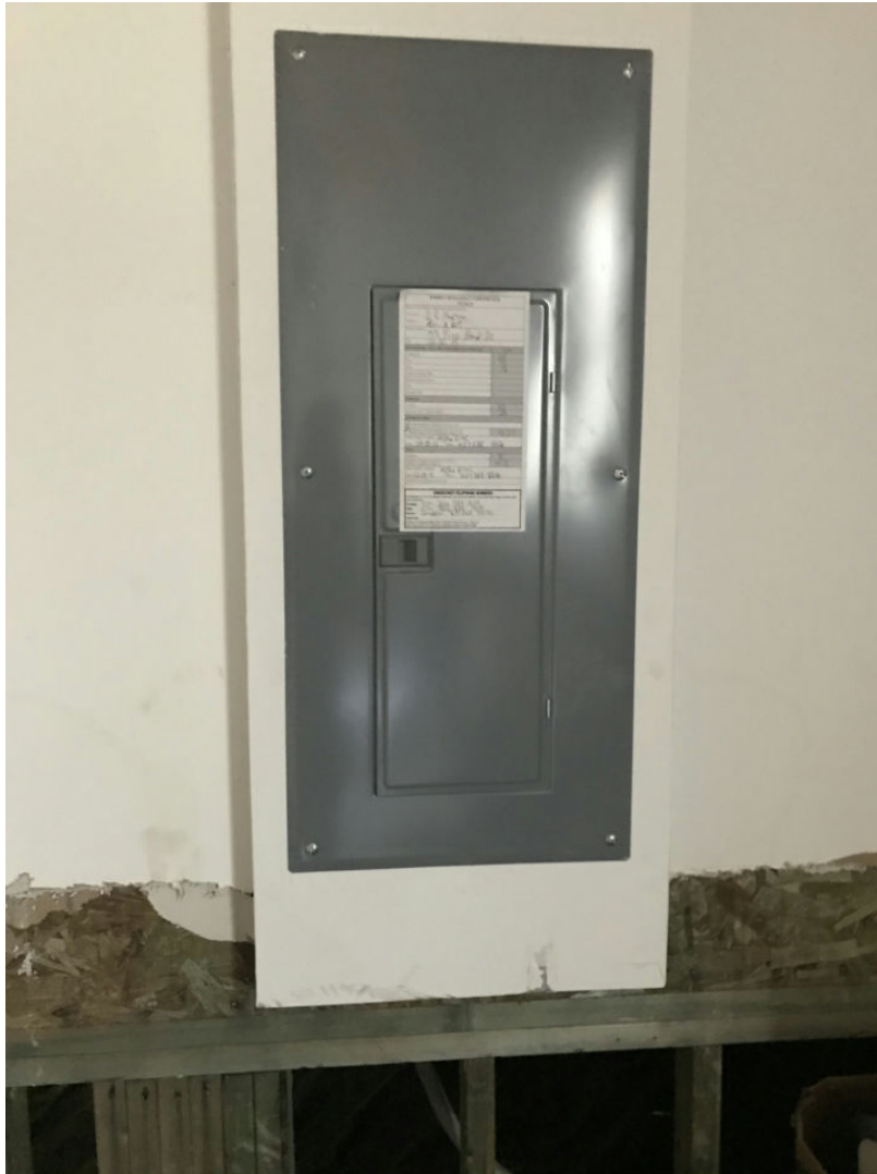
30 Main Level/Garage - 38-Garage (8) Date Taken: 7/1/2019
