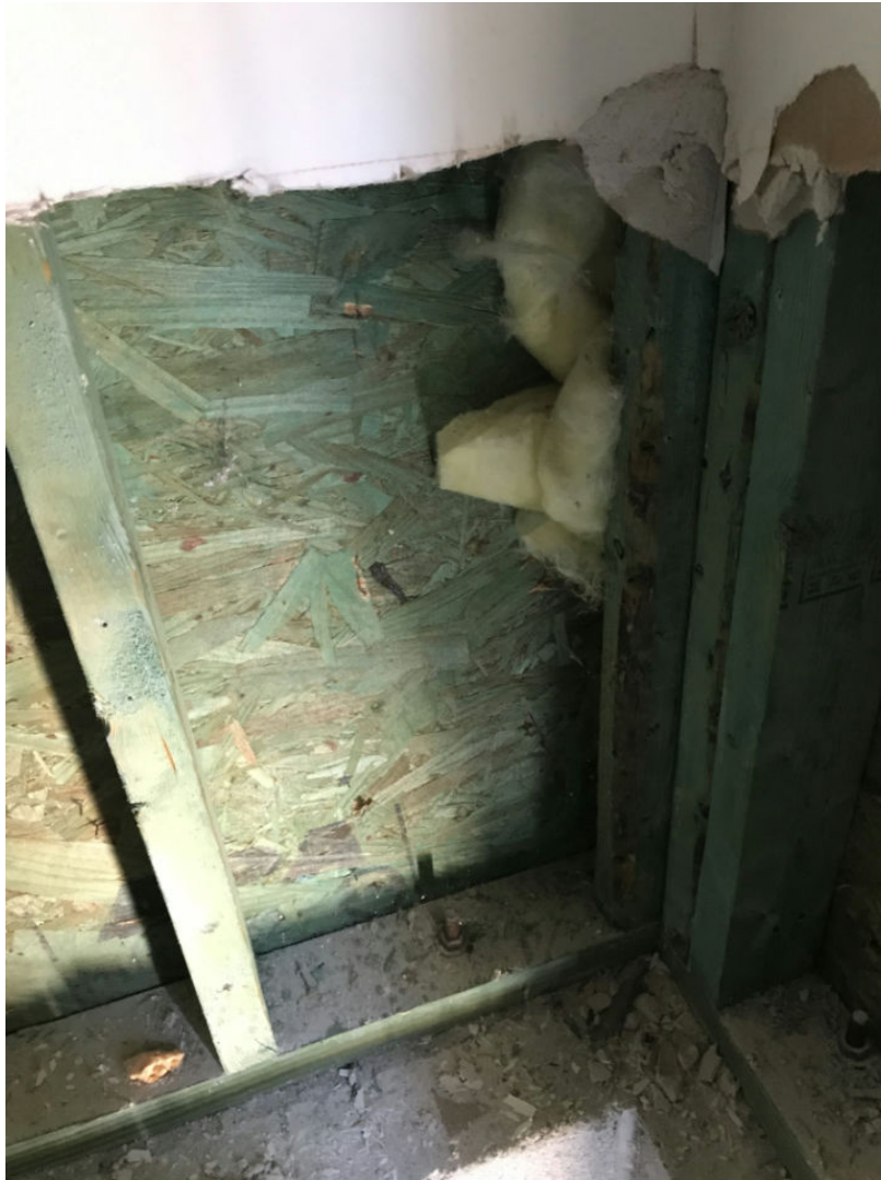
32 Main Level/Garage - 40-Garage Date Taken: 7/1/2019 (10)
