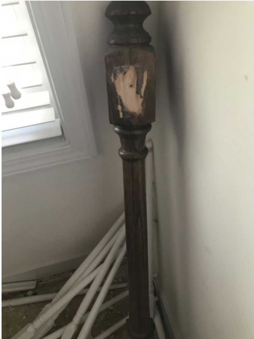
38 Main Level/Stairs1 - 46-Stairs (4) Date Taken: 7/1/2019
