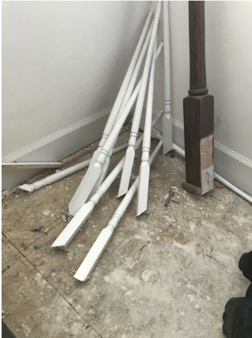
40 Main Level/Stairs1 - 48-Stairs (6) Date Taken: 7/1/2019
