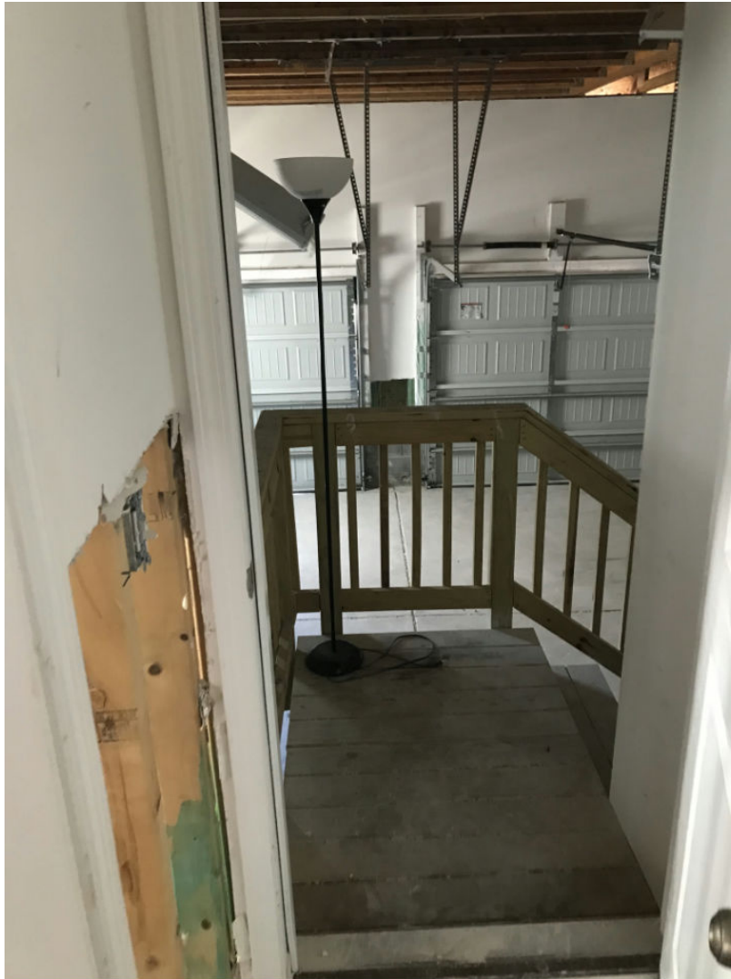
34 Main Level/Garage - 42-Garage Date Taken: 7/1/2019 (12)
