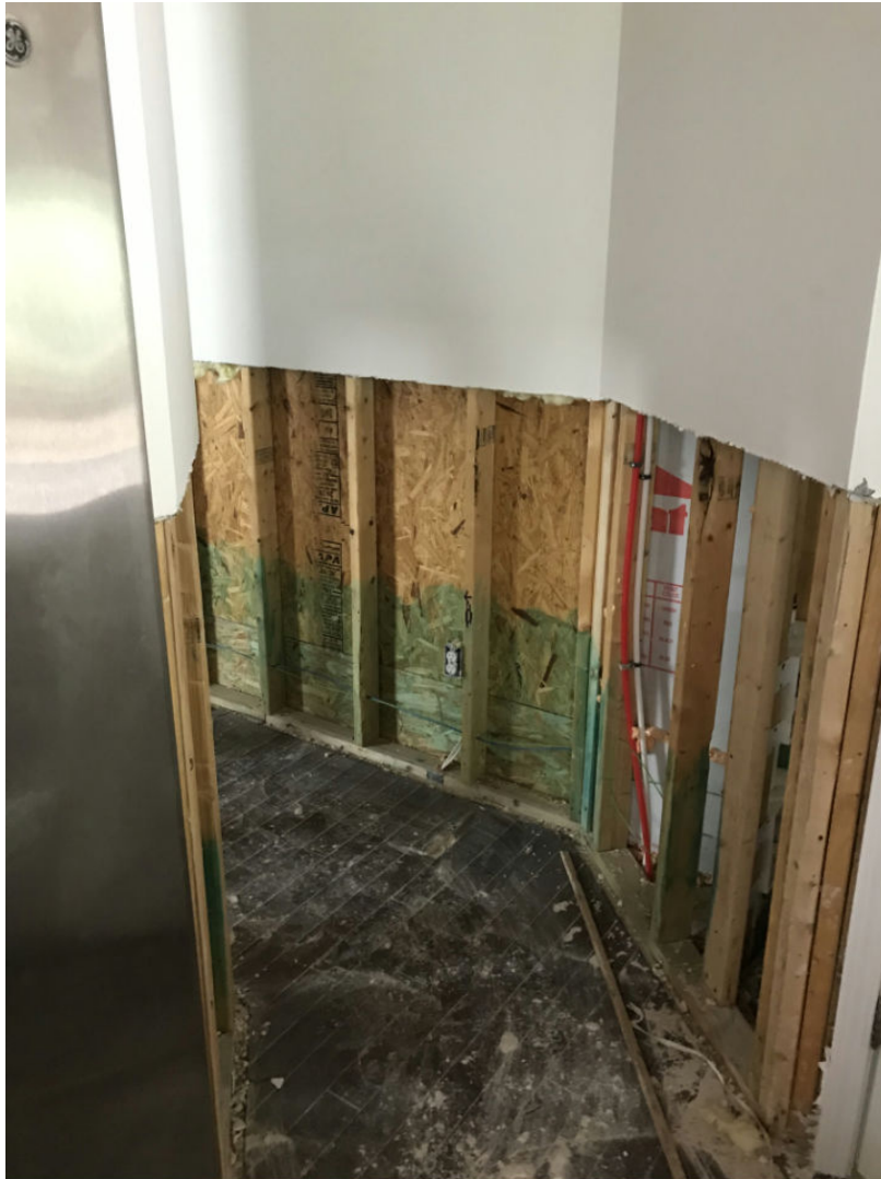
22 Main Level/Hallway2 - 31-Hallway Date Taken: 7/1/2019 1 (2)
