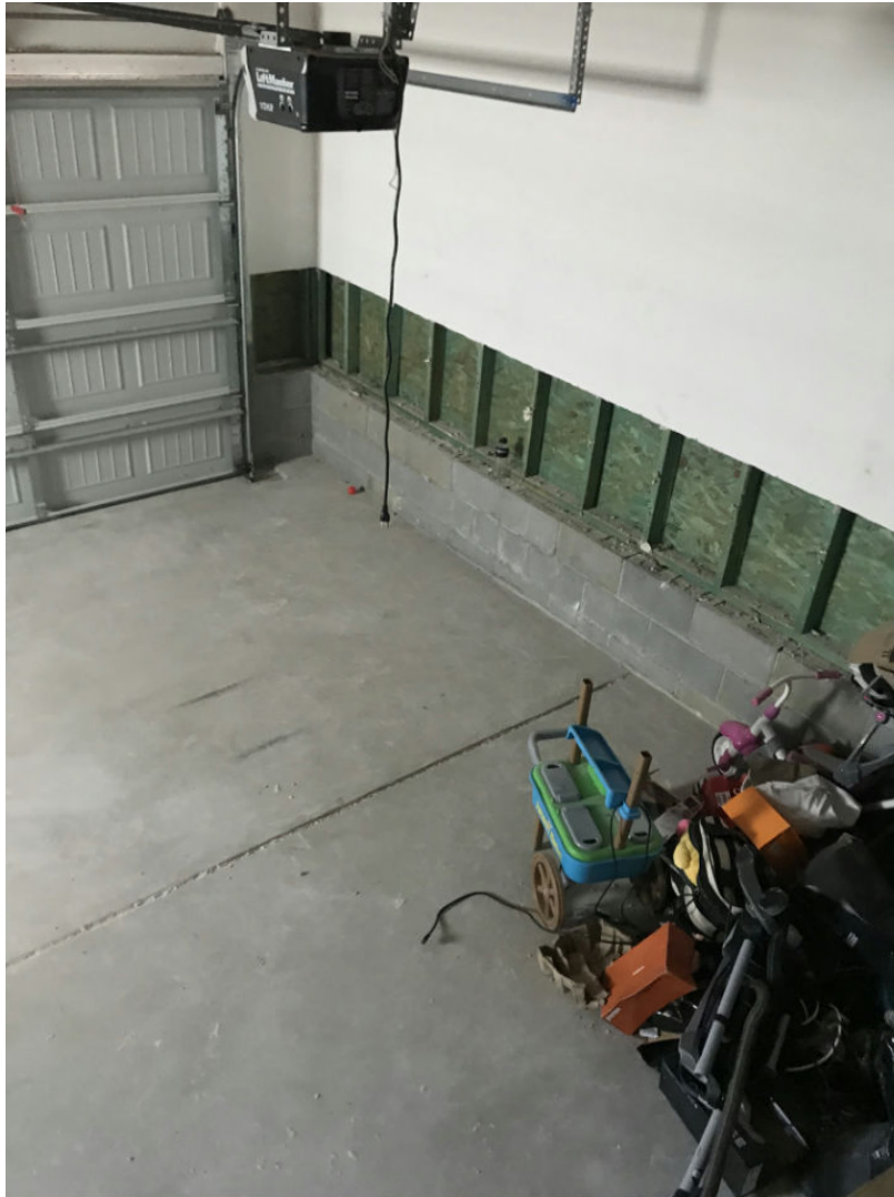
35 Main Level/Garage - 43-Garage (1) Date Taken: 7/1/2019
