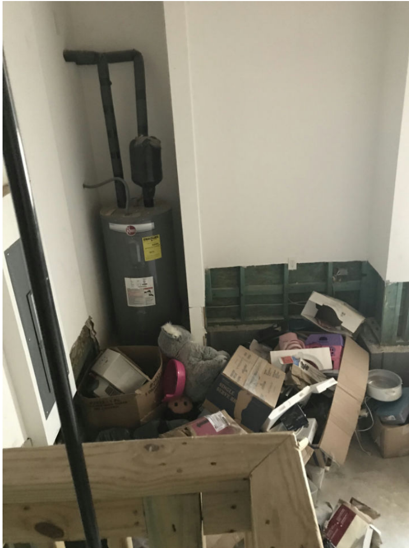
25 Main Level/Garage - 33-Garage (3) Date Taken: 7/1/2019
