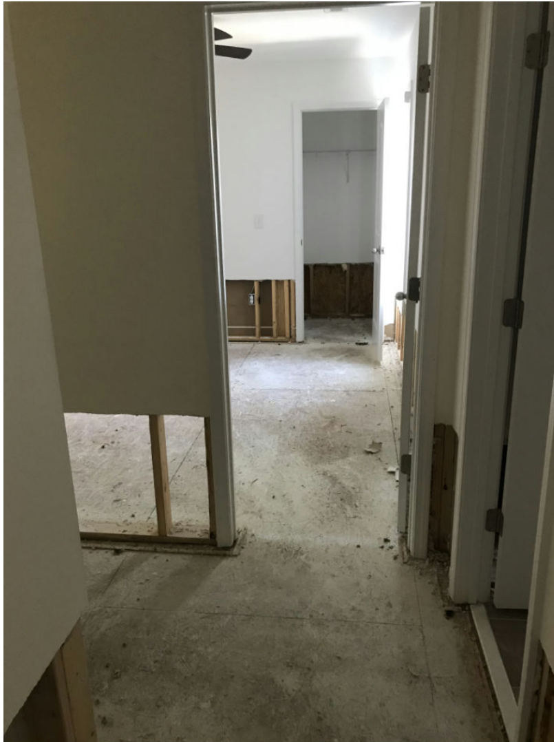
79 Upstairs/Hallway - 88-Hallway2 (2) Date Taken: 7/1/2019
