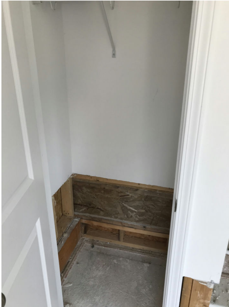
69 Upstairs/Storage - 78-Storage Date Taken: 7/1/2019
