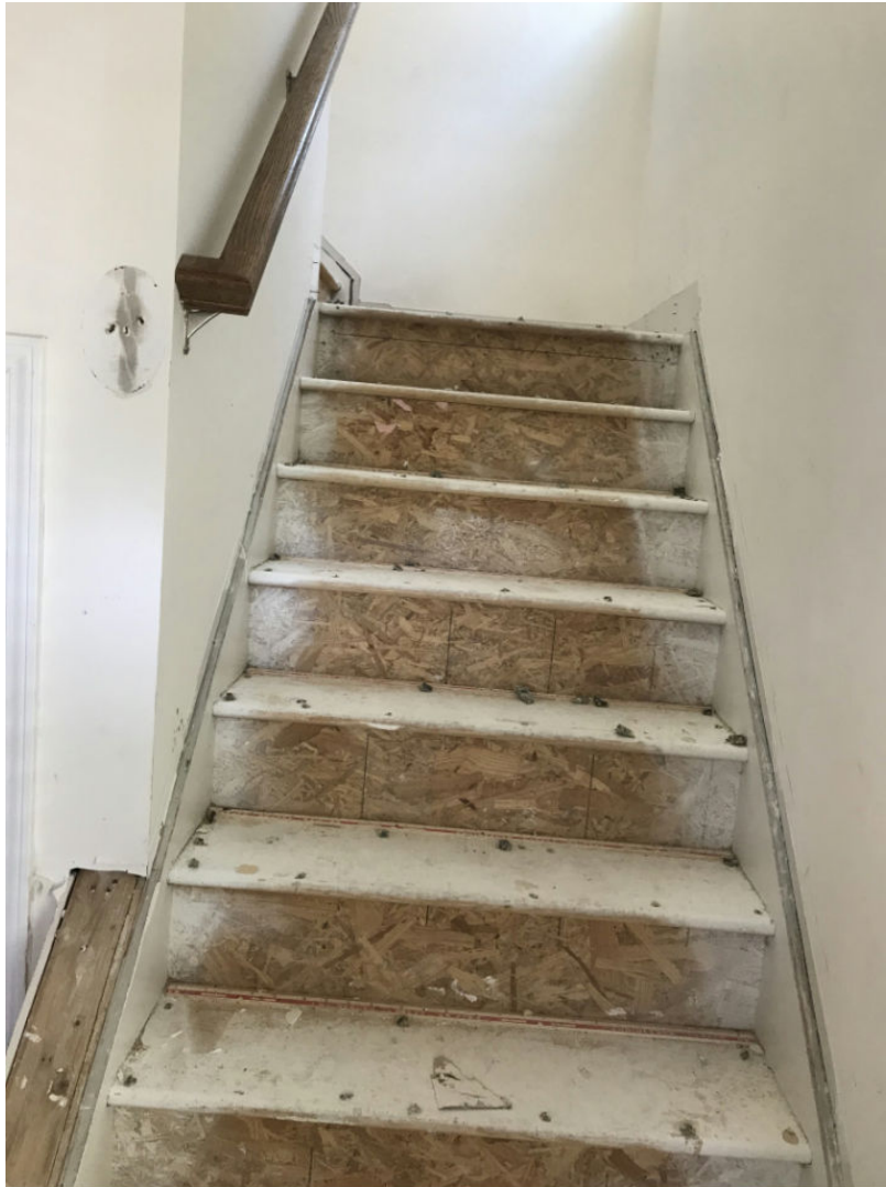
42 Main Level/Stairs1 - 50-Stairs (2) Date Taken: 7/1/2019
