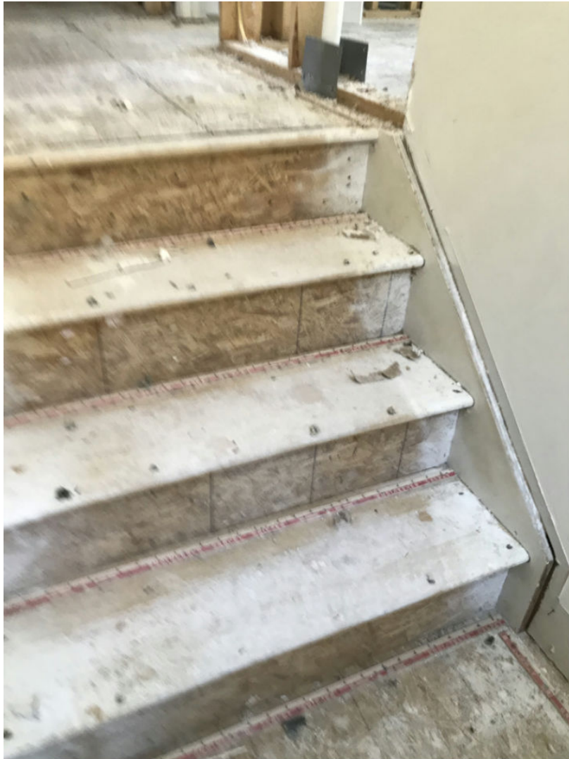
37 Main Level/Stairs1 - 45-Stairs (3) Date Taken: 7/1/2019
