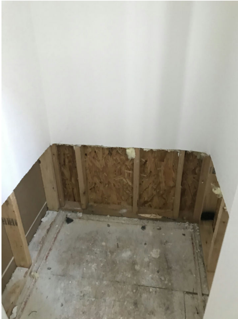
58 Upstairs/Closet 1 - 66-Clst1 (2) Date Taken: 7/1/2019
