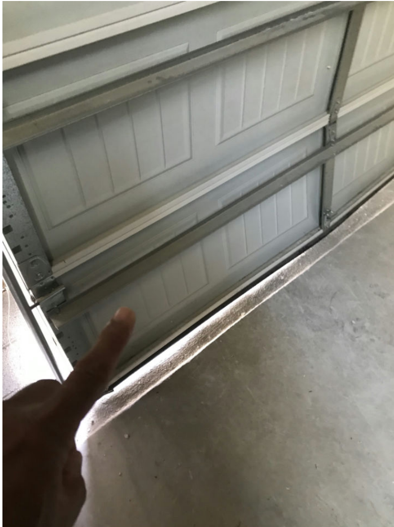
26 Main Level/Garage - 34-Garage (4) Date Taken: 7/1/2019
