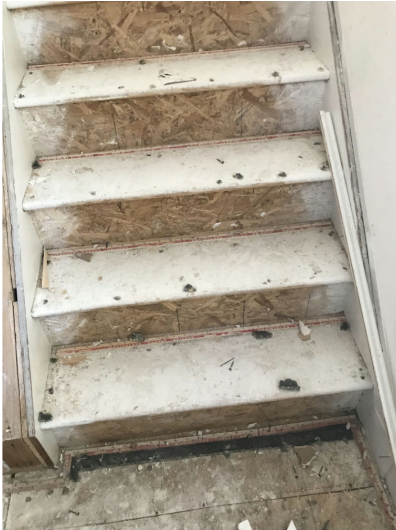
41 Main Level/Stairs1 - 49-Stairs (1) Date Taken: 7/1/2019
