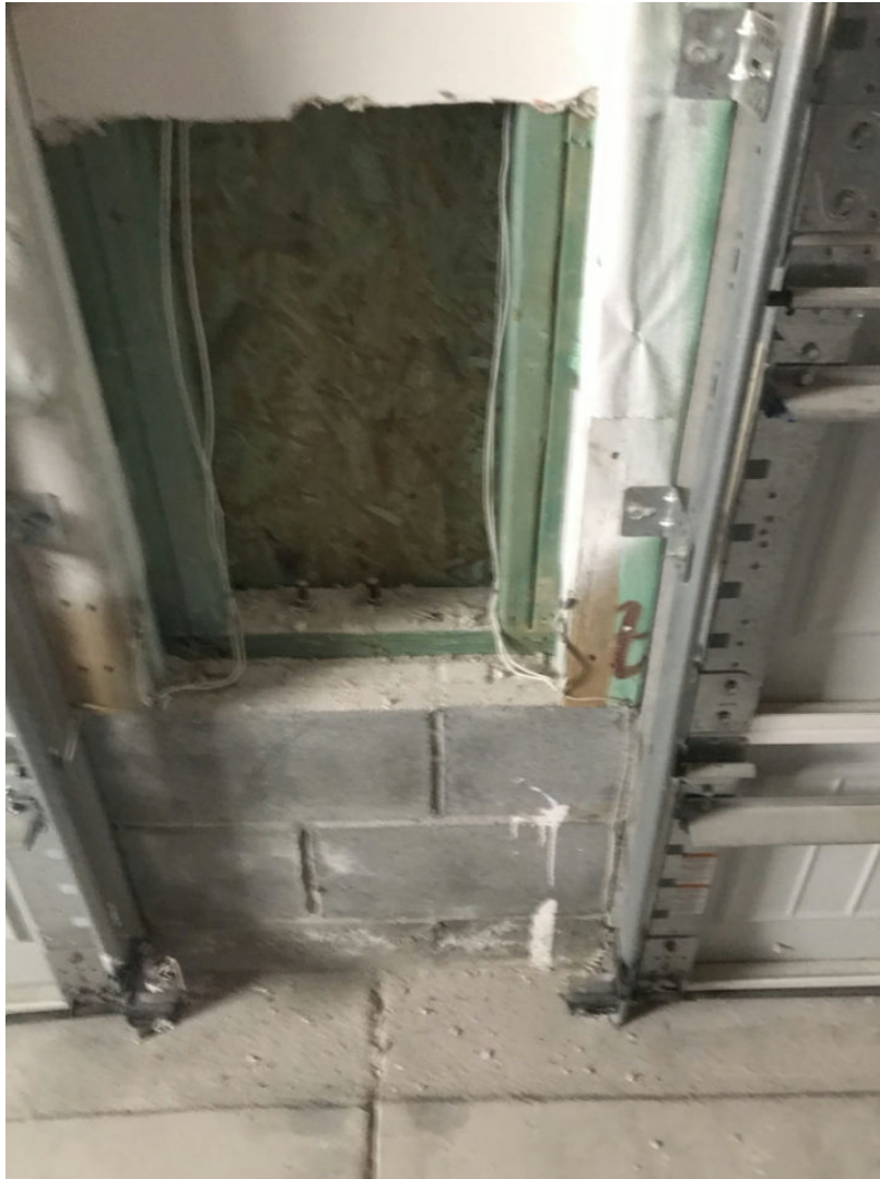
33 Main Level/Garage - 41-Garage Date Taken: 7/1/2019 (11)
