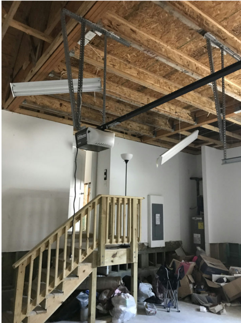
28 Main Level/Garage - 36-Garage (6) Date Taken: 7/1/2019
