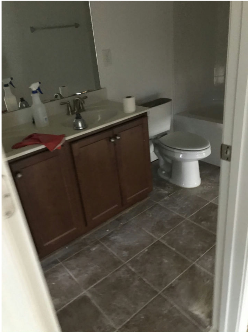
75 Upstairs/Bathroom - 84-Bathroom Date Taken: 7/1/2019 (2)
