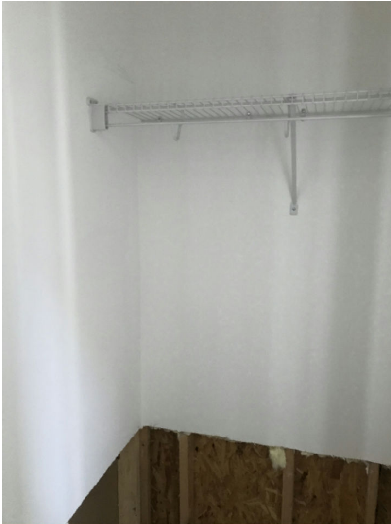
57 Upstairs/Closet 1 - 65-Clst1 (1) Date Taken: 7/1/2019
