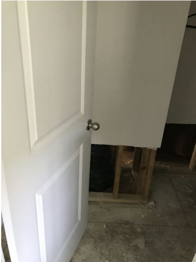
48 Upstairs/MasterW.C - 56-W.C (2) Date Taken: 7/1/2019
