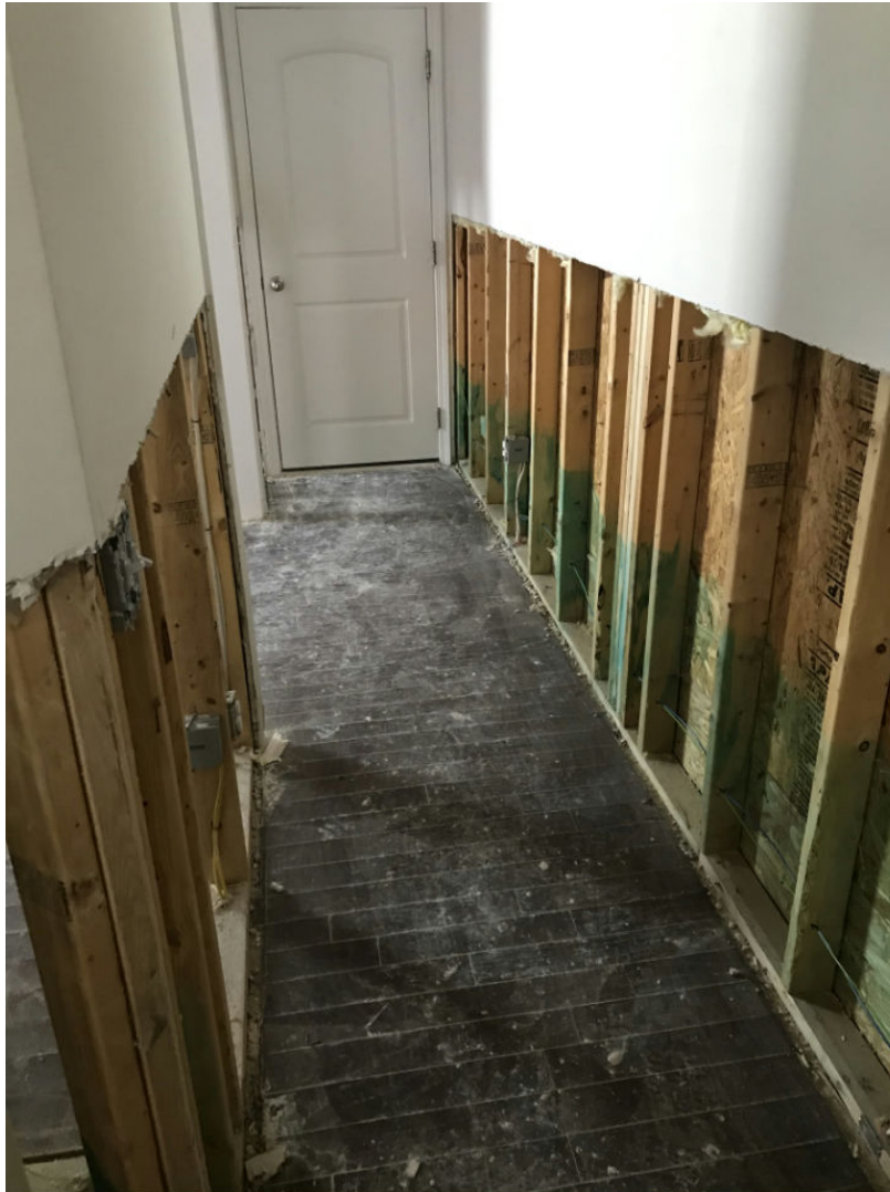
23 Main Level/Hallway2 - 32-Hallway Date Taken: 7/1/2019 1 (3)
