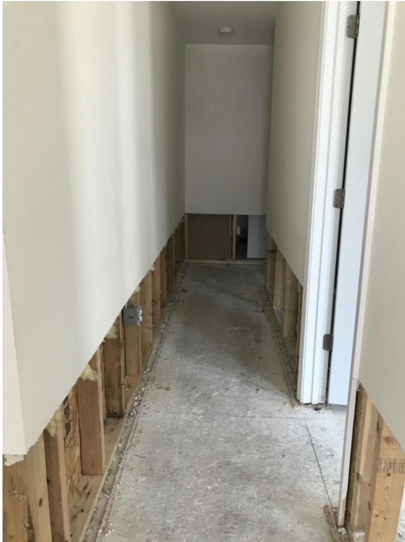
78 Upstairs/Hallway - 87-Hallway2 (1) Date Taken: 7/1/2019
