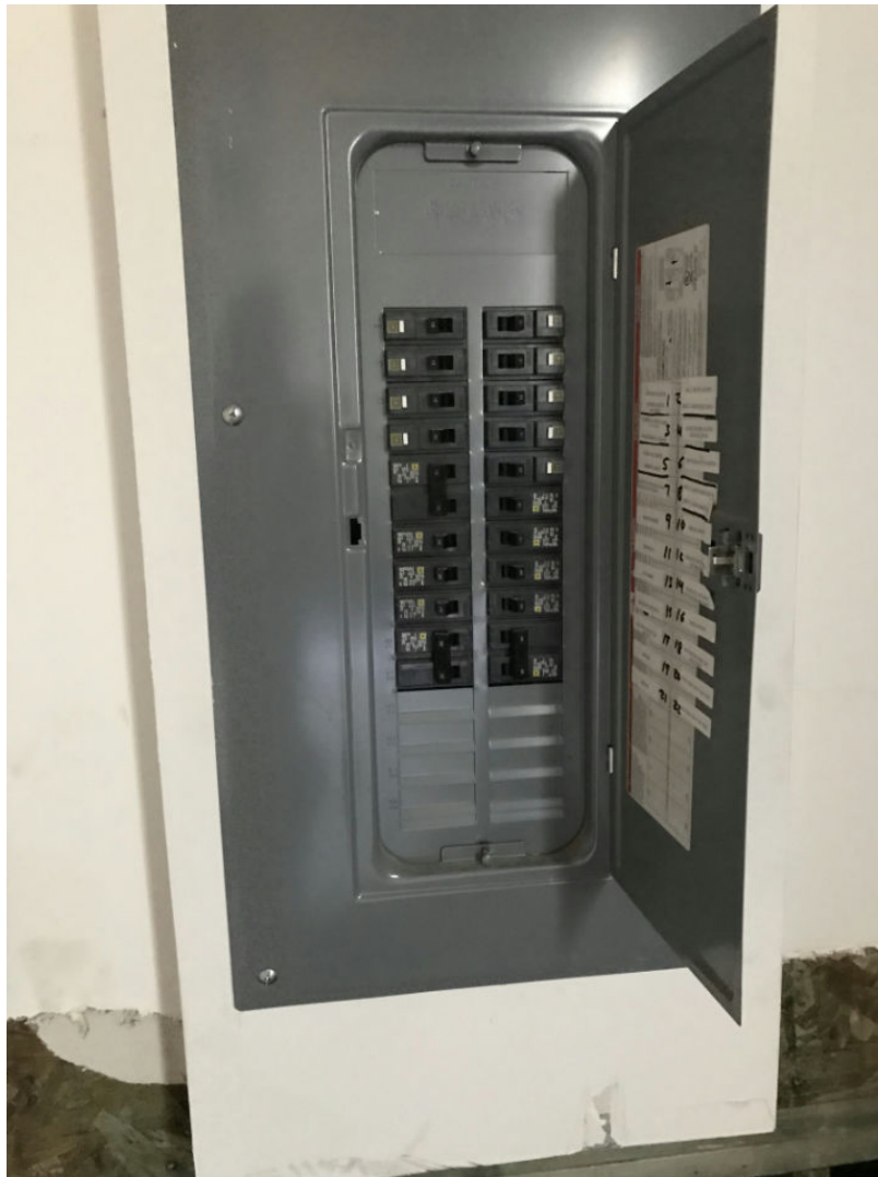
31 Main Level/Garage - 39-Garage (9) Date Taken: 7/1/2019
