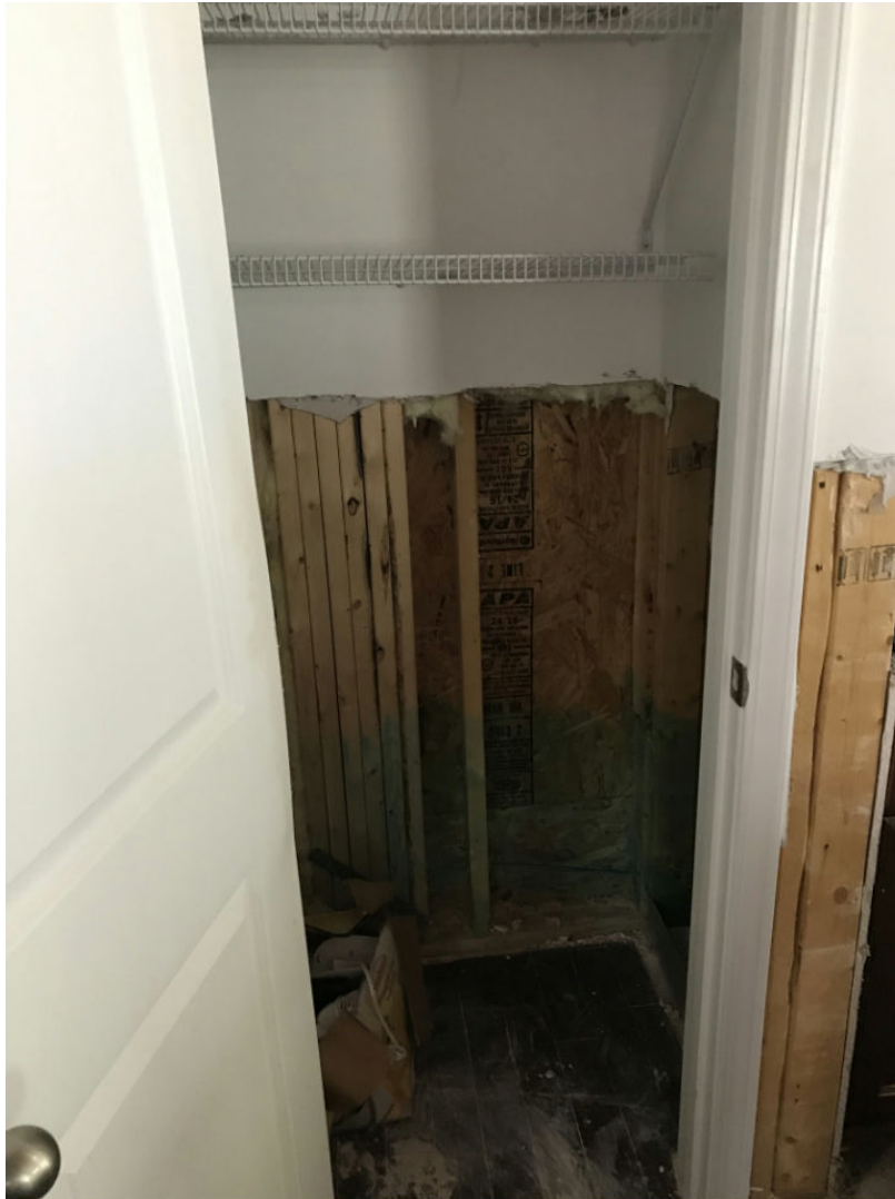
17 Main Level/Pantry - 26-Pantry Date Taken: 7/1/2019
