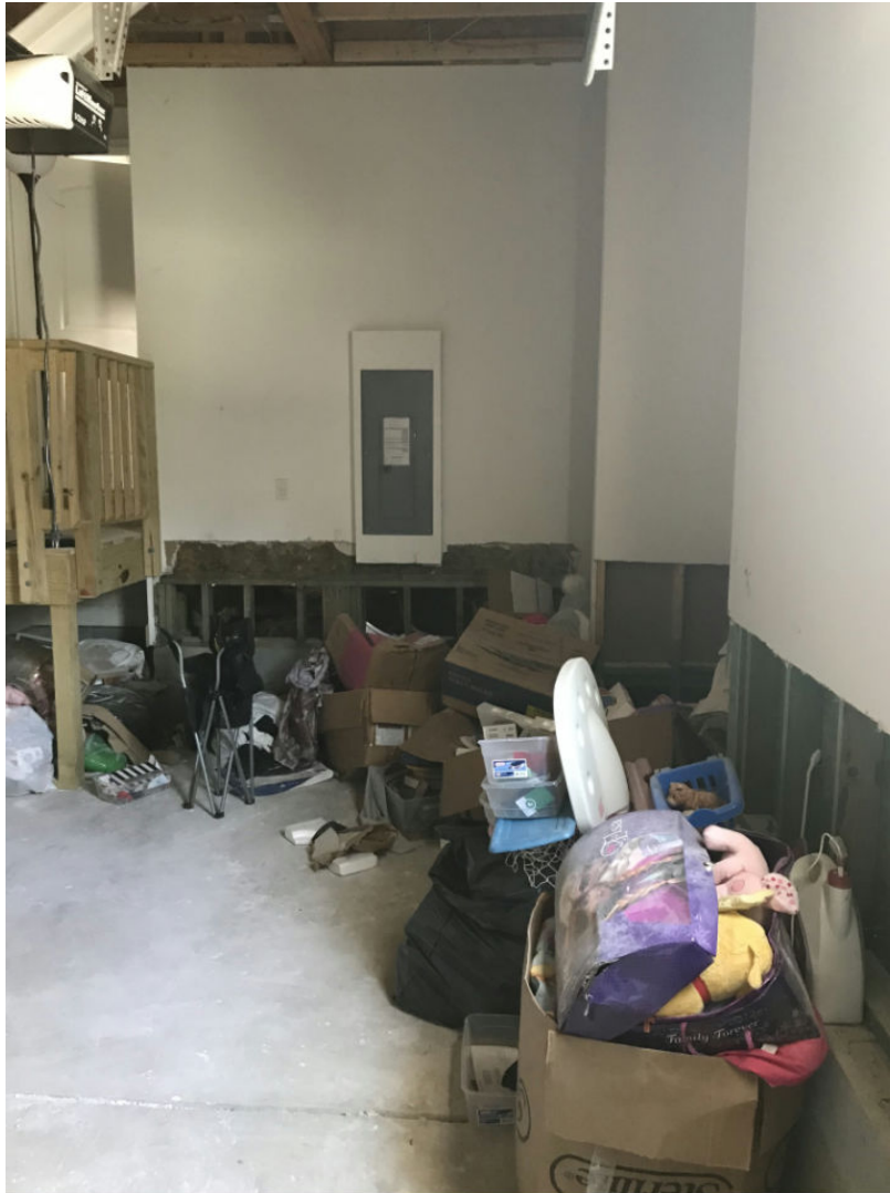
27 Main Level/Garage - 35-Garage (5) Date Taken: 7/1/2019
