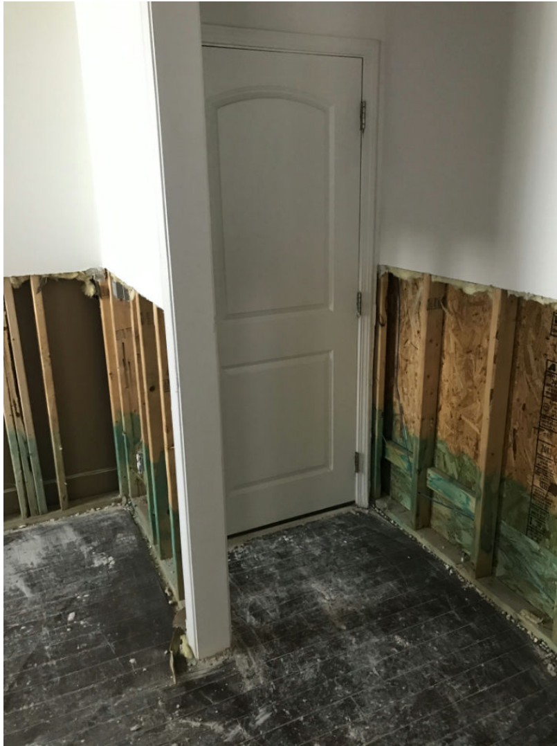
21 Main Level/Hallway2 - 30-Hallway Date Taken: 7/1/2019 1 (1)
