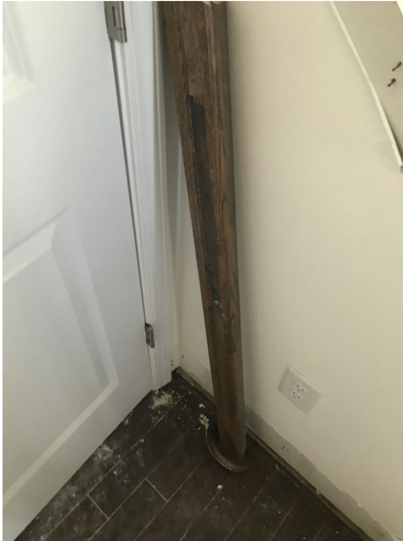
39 Main Level/Stairs1 - 47-Stairs (5) Date Taken: 7/1/2019
