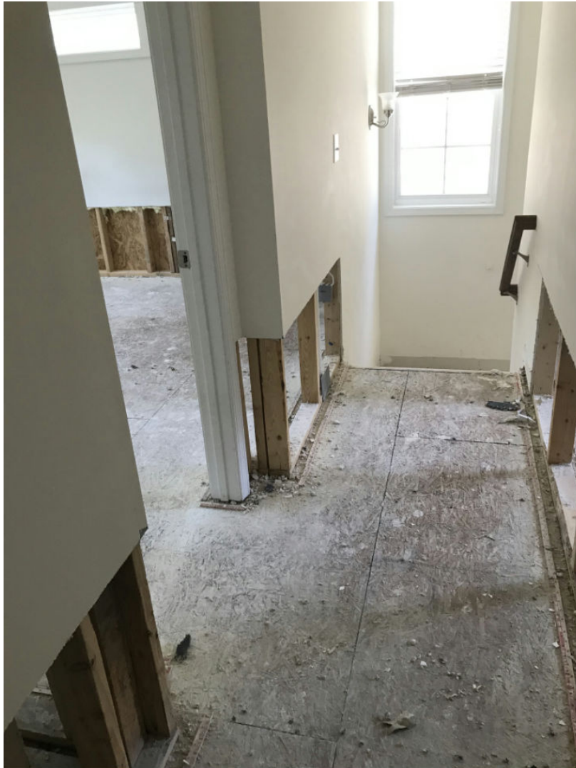
81 Upstairs/Hallway - 90-Hallway2 (4) Date Taken: 7/1/2019
