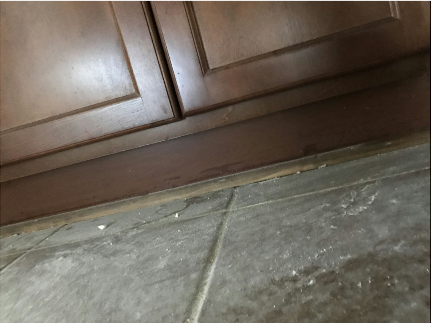
74 Upstairs/Bathroom - 83-Bathroom Date Taken: 7/1/2019 (1)
