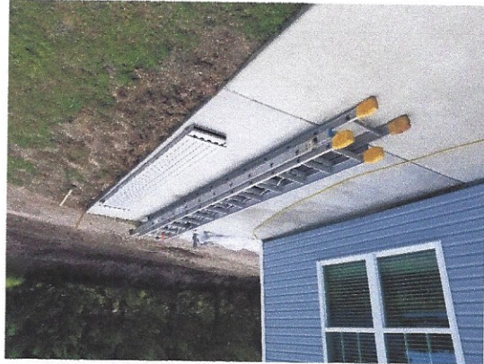
Picture 3 – Example of new porch slab
