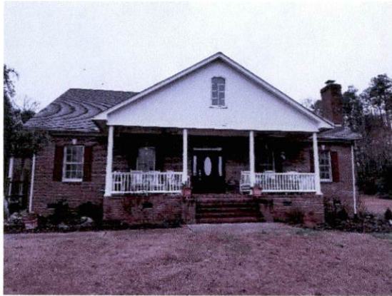
Picture 1 – 2755 Brick Mill Road, Lillington, NC
