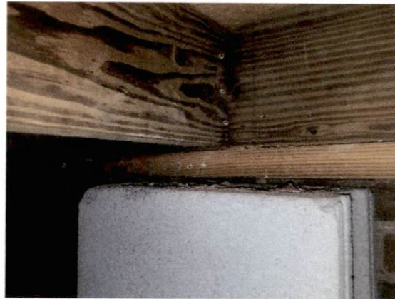
Picture 10 – Example of out-of-contact masonry support
