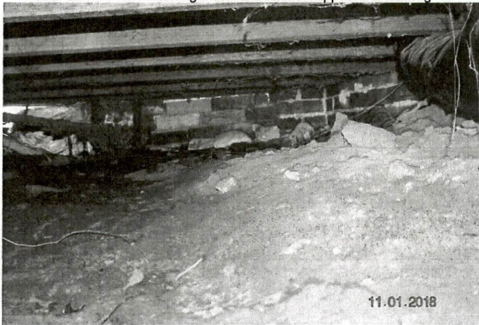
Photograph No. 24 – This photo is taken from the front looking to the right side of the rear wall. The face wall along the rear is damaged.
