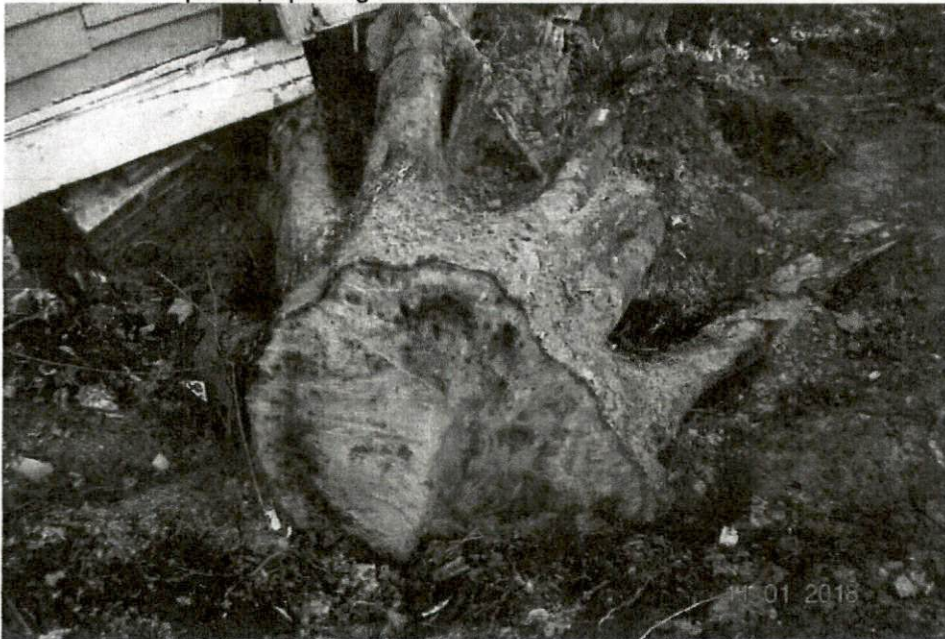
Photograph No. 3 – This is the left rear corner of the home. The tree fell toward the left in this photo, uplifting the left rear corner of the home.
