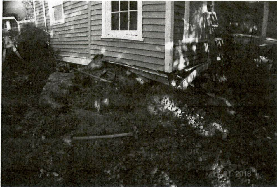
Photograph No. 3 – This is the left rear corner of the home. The tree fell toward the left in this photo, uplifting the left rear corner of the home.
