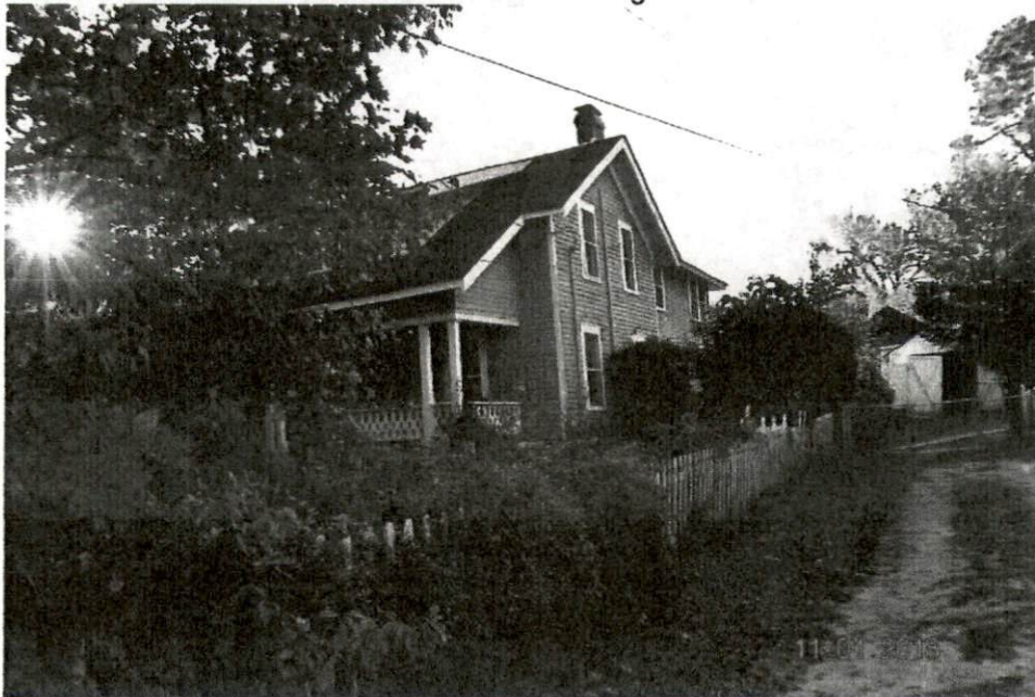
Photograph No. 2 – A view of the home from the right front.
