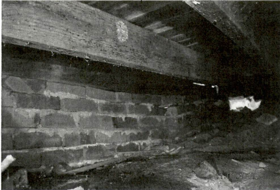
Photograph No. 20 – ... but the face wall is not. The face wall is not a structural component.
