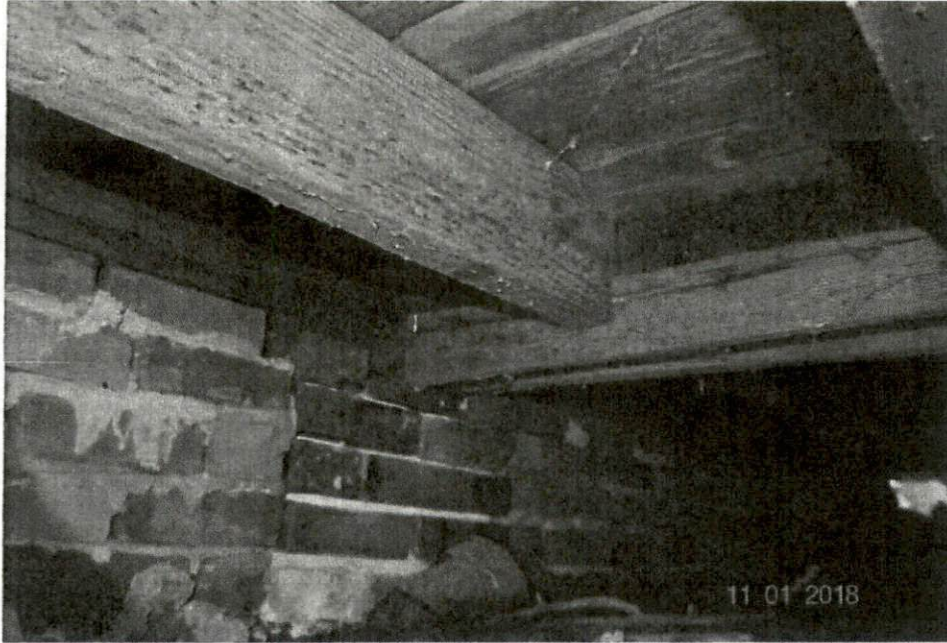
Photograph No. 19 – The pier supporting the left-to-right girder on the left wall is in good shape...
