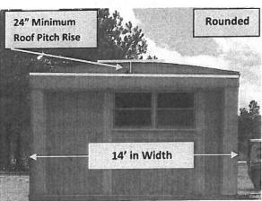
Note: Most Rounded Roofs **Will Not** Meet The Roof Pitch Requirement As Illustrated. The Measurement From The Peak Of The Roof To The Base Line Of The Roof Must Be 12" For Every 7' Of Total Width Of The Home. (Ex: 14' Wide Home = 24" Roof Rise)
